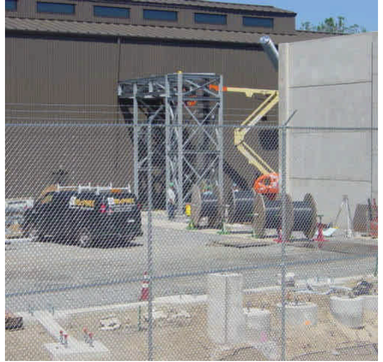
Electrical connection and tie-in work continues inside the substation. Crews were on-site preparing to pull cable.
