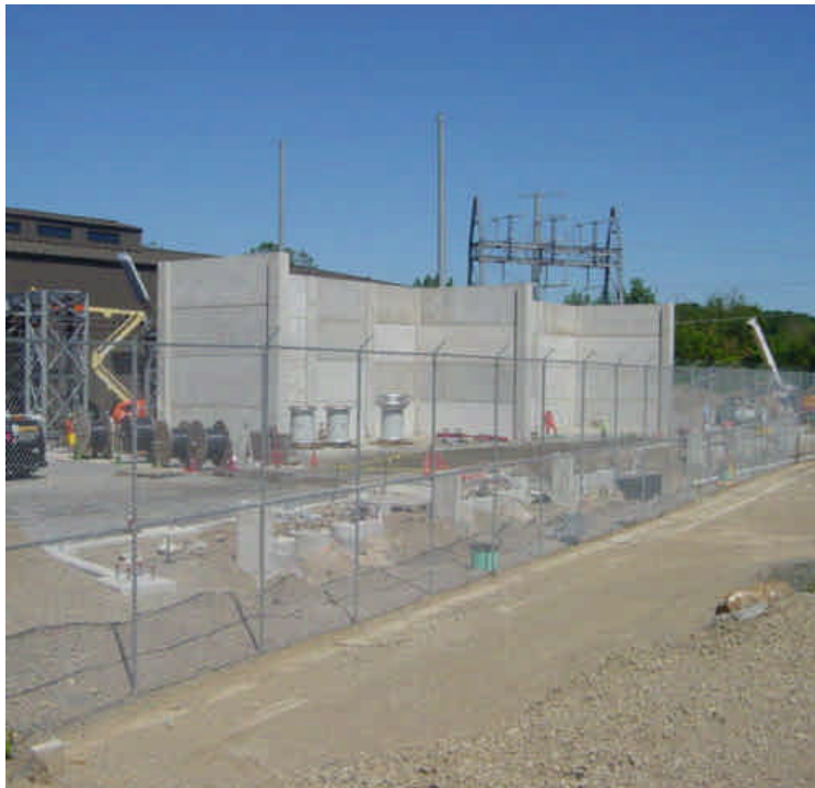
Minor excavation work was underway inside the substation.
