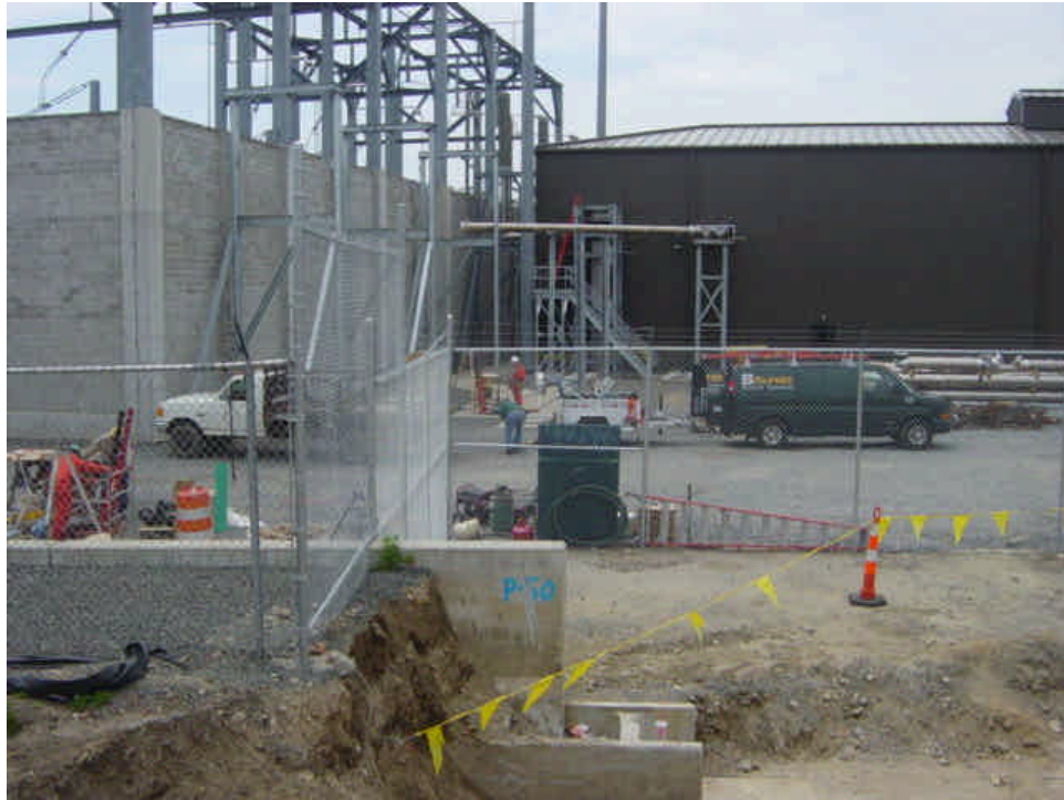
Electrical contractors were on site proofing lines and pulling cables.
