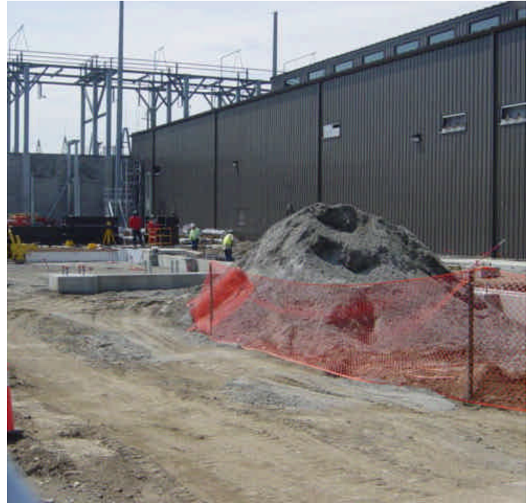
Trenching and earthwork continue within the Norwalk substation to accommodate the new 345-kV equipment. Foundations have already been installed. The photo on the right shows a soil stockpile that was observed without adequate containment. However, the pile appeared to be actively used.
