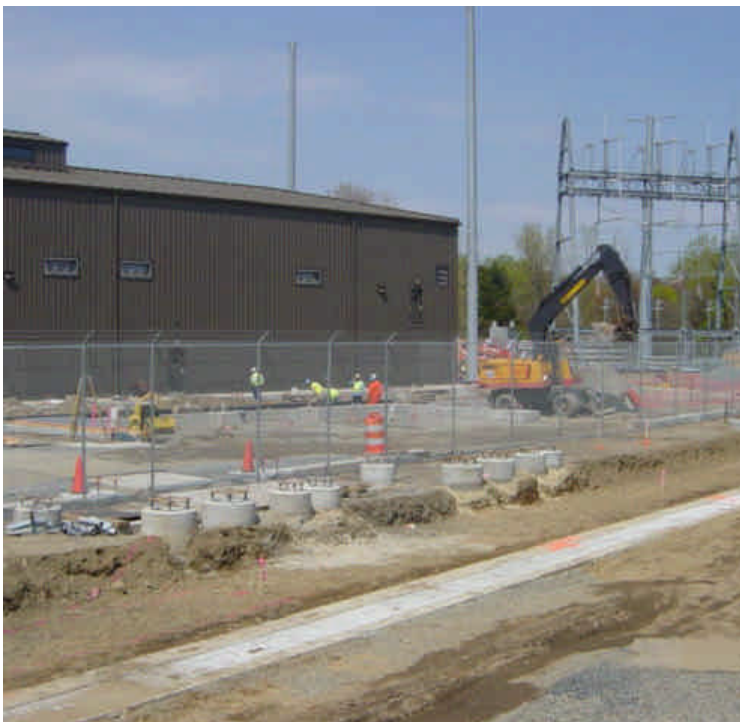
Foundations have been installed to accommodate the new 345-kV equipment within Norwalk substation. The chain link perimeter fence has been relocated to accommodate this work. The modular concrete retaining wall has been temporarily removed to accommodate trenching and tie-in activities.
