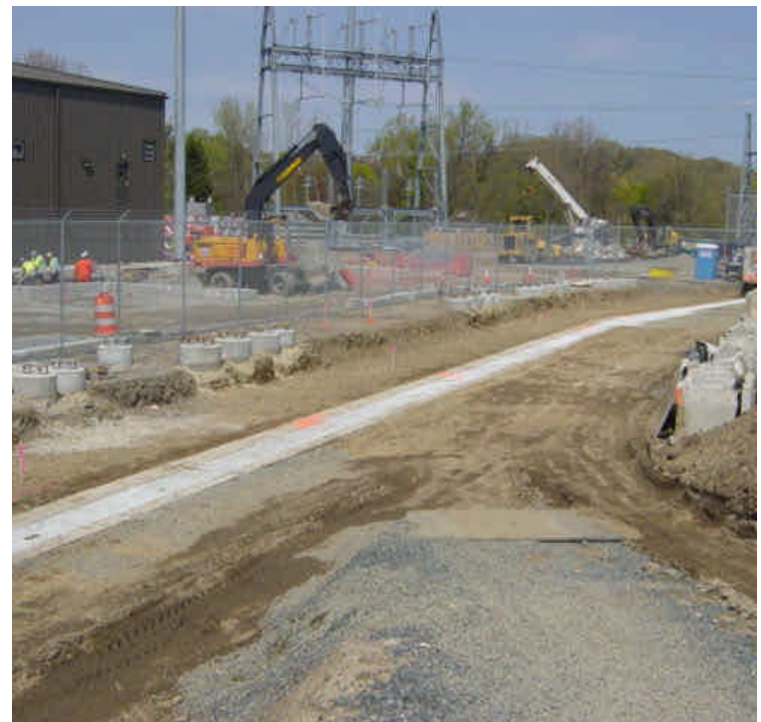
Foundations have been installed to accommodate the new 345-kV equipment within Norwalk substation. The chain link perimeter fence has been relocated to accommodate this work. The modular concrete retaining wall has been temporarily removed to accommodate trenching and tie-in activities.
