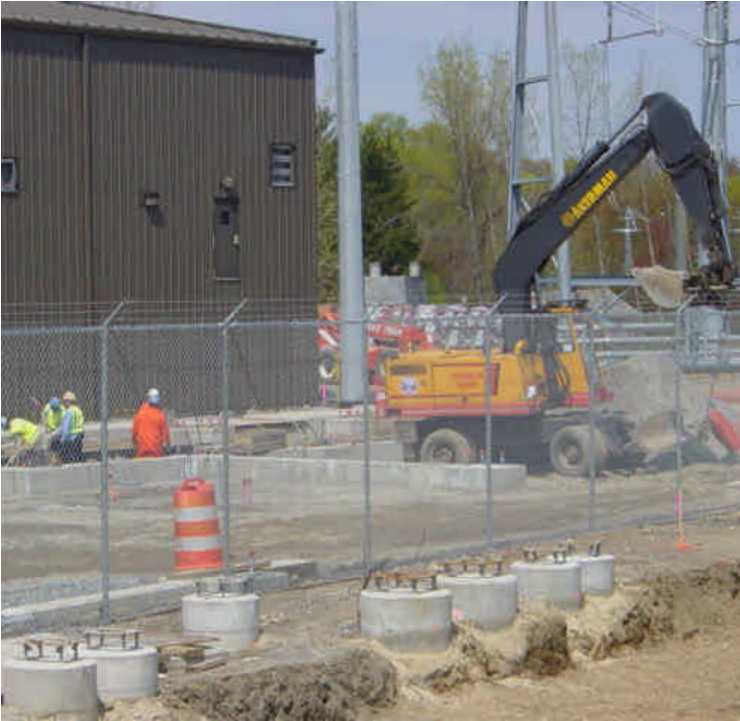
Trenching and earthwork continue within the Norwalk substation to accommodate the new 345-kV equipment. Foundations have already been installed. The photo on the right shows a soil stockpile that was observed without adequate containment. However, the pile appeared to be actively used.
