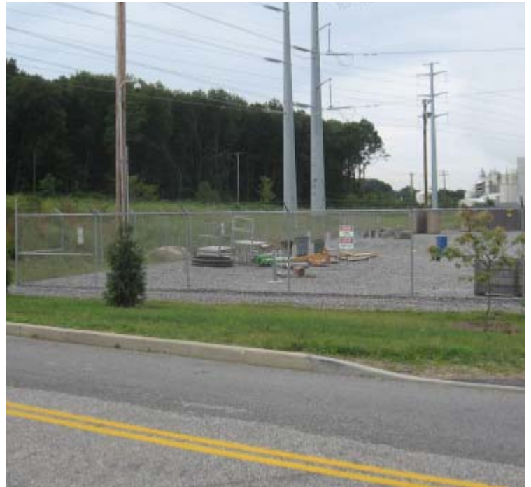
East Devon Substation: A general view of the NE corner of the substation and ROW.
