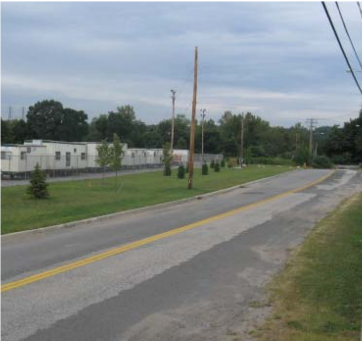
East Devon Substation: A view of Plains Rd. No sediment tracking was observed.
