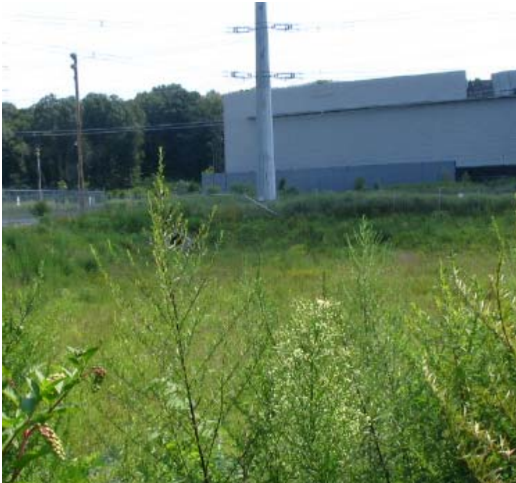
East Devon Substation: The retention basin is approximately 70-80% vegetated.
