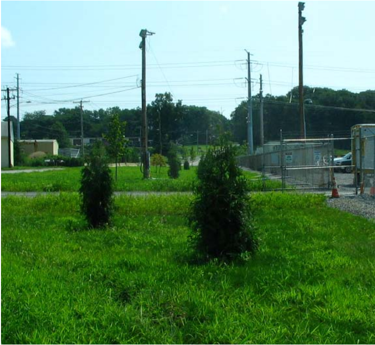
East Devon Substation: A view of vegetation growth along Plains Rd.
