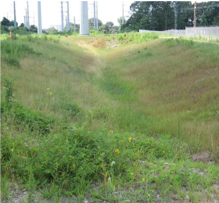
East Devon Substation: The southern section of the vegetated swale is stabilized with 90% vegetative cover.
