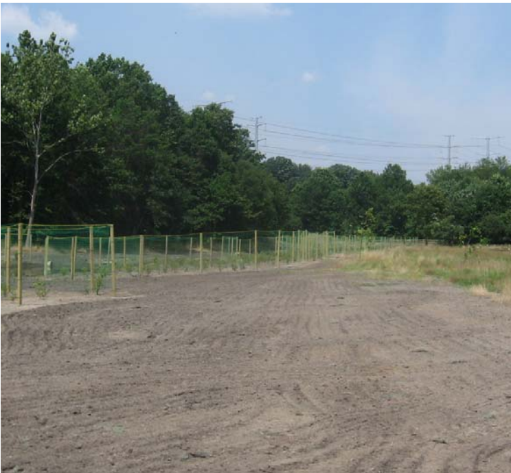
Wetland Mitigation Area: A view of the plantings/deer fencing along the eastern side of the mitigation area.
