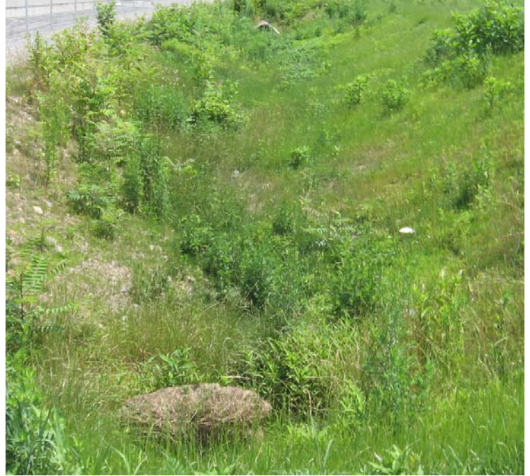
East Devon Substation: A view of the middle section of the vegetated swale.
