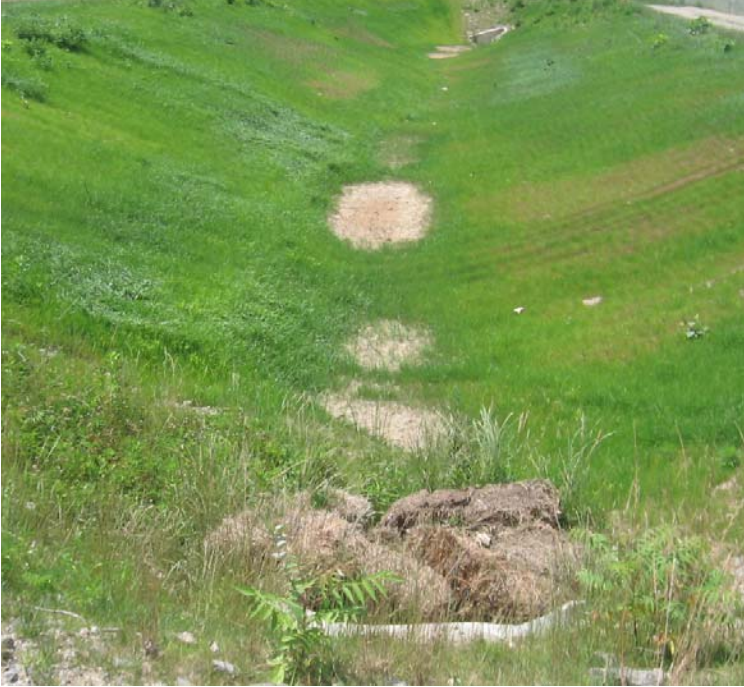
East Devon Substation (Milford): A view of the southern section of the vegetated swale.
