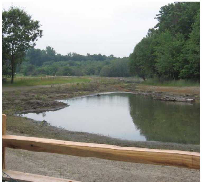
Wetland Mitigation Area (Eisenhower Park): A view of a portion of the mitigation area. Exposed soils remain stable, and the plantings appear to be doing well at this time.
