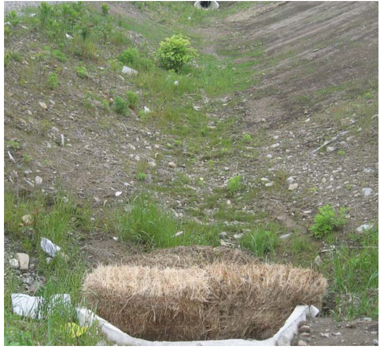
East Devon Substation: A view of the central portion of the vegetated swale. Soils appear stable and vegetation growth has been noted.
