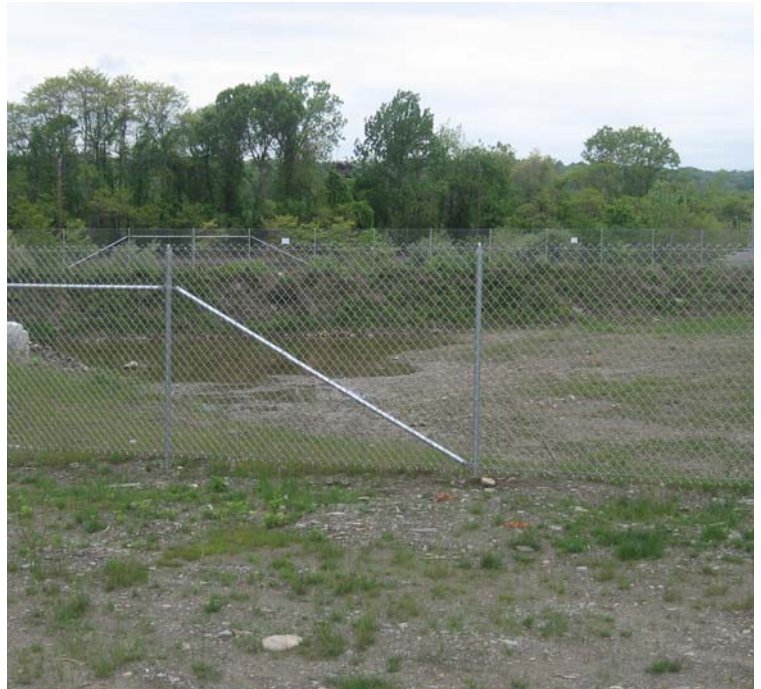
East Devon Substation: A view of the detention basin. Some grass growth has been observed.
