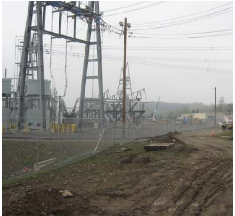
East Devon Substation: An additional view of construction at the substation.
