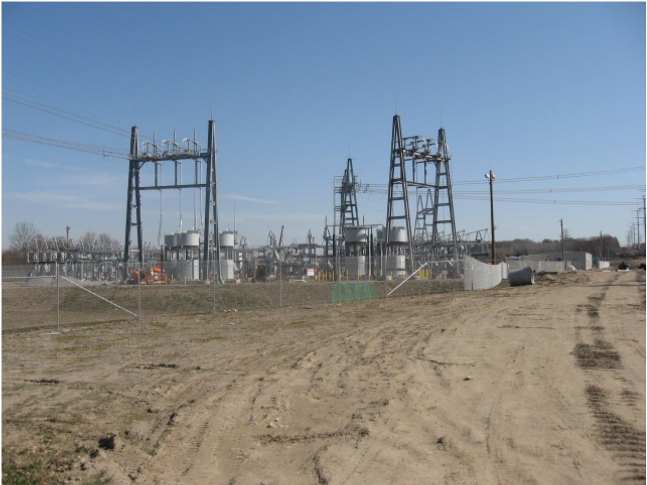
East Devon Substation (Milford): A general view of substation construction.
