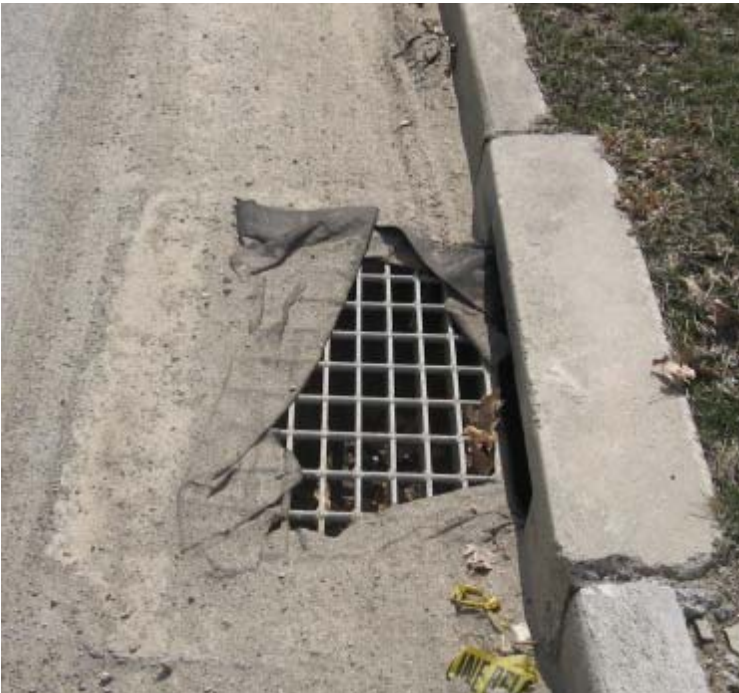
East Devon Substation (Plains Rd): “Silt saks” remain installed within the catch basins located in this area. Inlet protection is not provided on Plains Rd.
