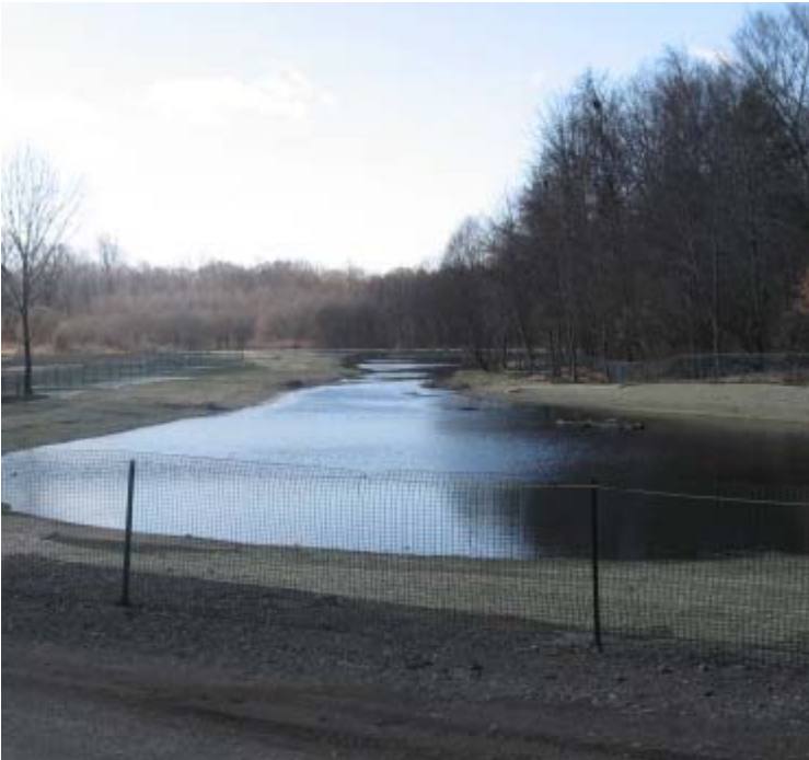
Eisenhower Park (Milford): A general view of the substation mitigation wetland.
