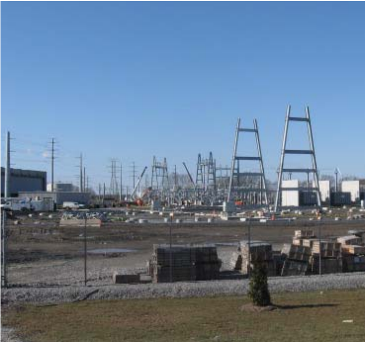
East Devon Substation (Milford): A general view of construction at the substation.
