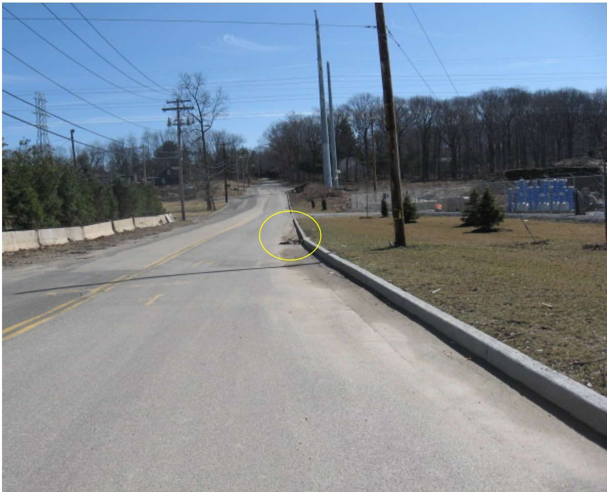
East Devon Subststion (Milford): Sediment has been removed from the "Silt Saks" along Plains Rd.
