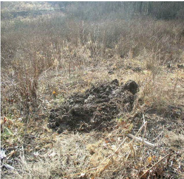
Accumulated sediment was removed from the wetlands and culvert across Carpenter Ln. and spread appropriately in an upland
