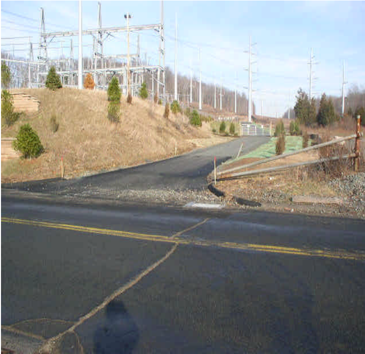
View along the eastern site access from Carpenter Lane. Some stone was migrating into the driveway from the 1A access point.
