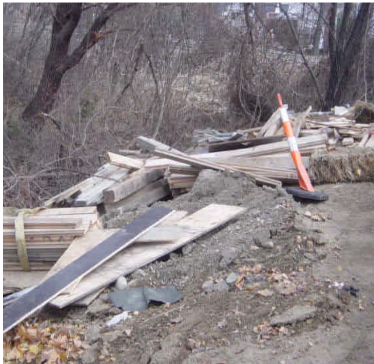
Haybales previously placed along the downgradient side of the slope near sta. #18 have been moved and no longer form a continuous barrier. Exposed soils remain. Materials were being stored in the area but it is unclear whether the lumber is project-related
