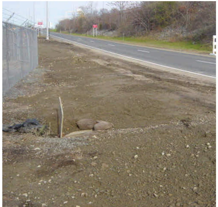
Existing drainage swale near sta. #5 (photo on left) appears to have run along the shoulder of the off ramp and drain into the inlet structure (photo on right). Trench work has altered the grades in this area and the drainage swale has not been reestablished. Inlet was protected, but sediment has still accumulated inside the structure. The drainage swale is not addressed in the D&M plan but efforts need to be made to ensure appropriate drainage. Exposed soils along the off-ramp have the potential to erode and need stabilization sufficient for winter months.
