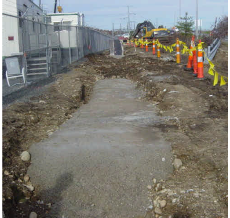
Flowable fill has been placed in the trench near sta. #5
