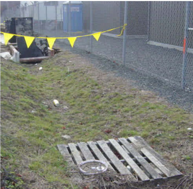
Existing drainage swale near sta. #5 (photo on left) appears to have run along the shoulder of the off ramp and drain into the inlet structure (photo on right). Trench work has altered the grades in this area and the drainage swale has not been reestablished. Inlet was protected, but sediment has still accumulated inside the structure. The drainage swale is not addressed in the D&M plan but efforts need to be made to ensure appropriate drainage. Exposed soils along the off-ramp have the potential to erode and need stabilization sufficient for winter months.
