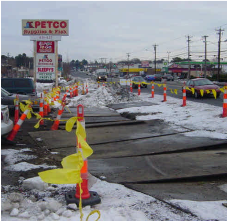
Vault tie-in work continues near sta. #144-146. Steel plates are in place.
