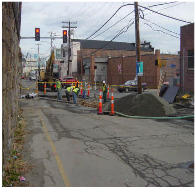
Trenching activities continue along Railroad Avenue near sta. #791-792.
