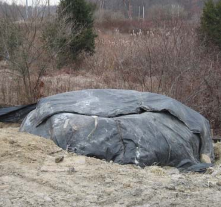
Eisenhower Park: Foundation work is complete at structure #24028. Controls remain intact.
