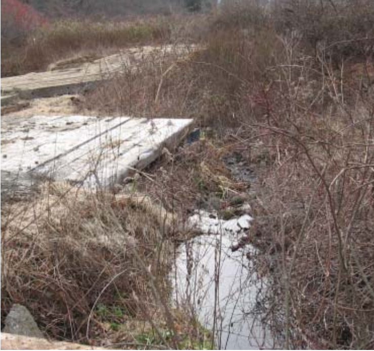
Rimmon Rd: Additional view of the crane pad/ stream.
