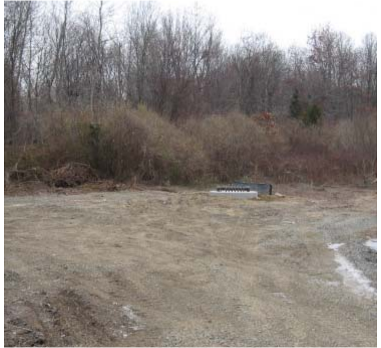
Eisenhower Park (Milford): Foundation work is complete at structure #24029.
