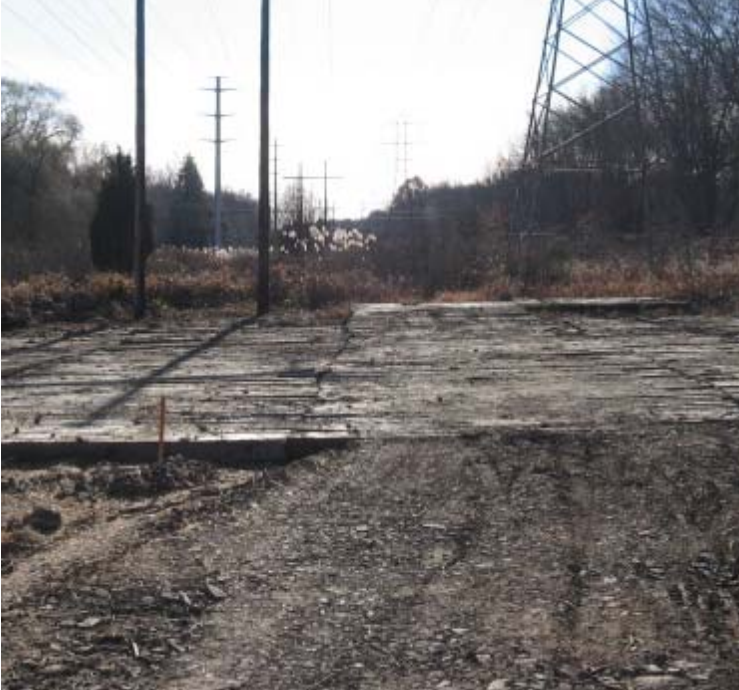
Manville Rd (Woodbridge): Pad reclamation is complete near structure 3915 and proposed structure 24102.
