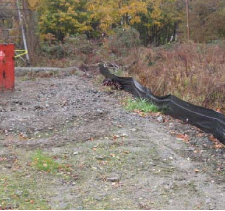
Oronoque Rd North (Milford): 345 kV foundation work is active in this area. Proper erosion controls are in place.
