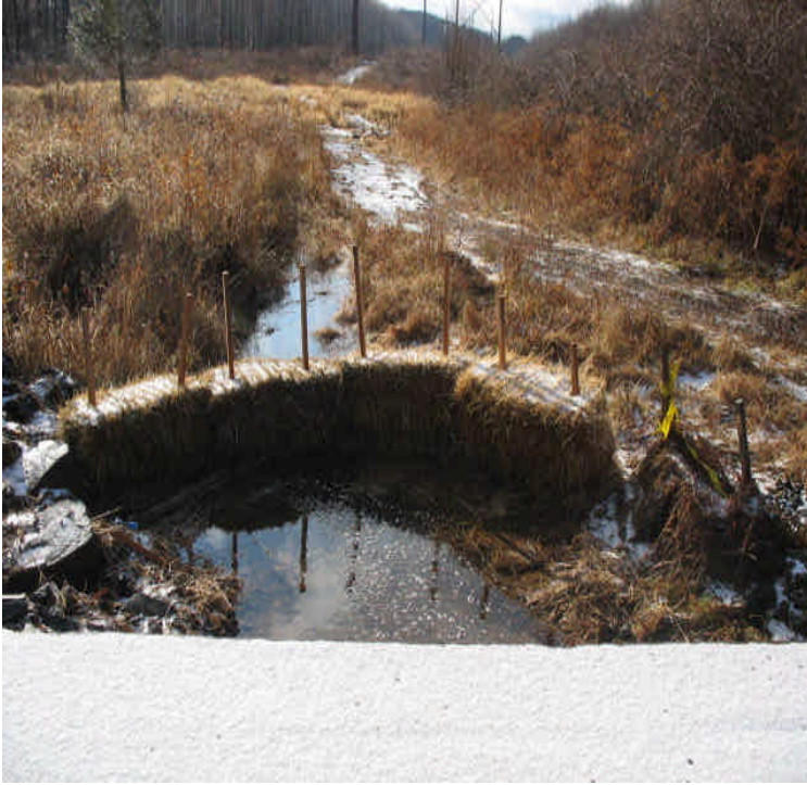
Carpenter Lane: New haybales remain at the wetland outlet. Previously accumulated sediment should be removed prior to restoration.
