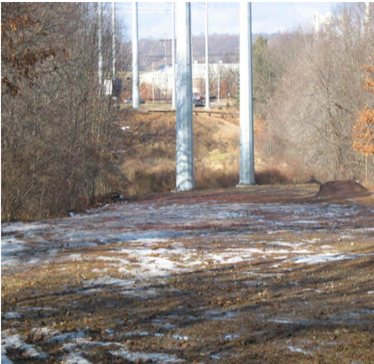
Docker Dr: Previously reclaimed area is also being disturbed by ATVs. Seed and mulch has washed away and should be reapplied.
