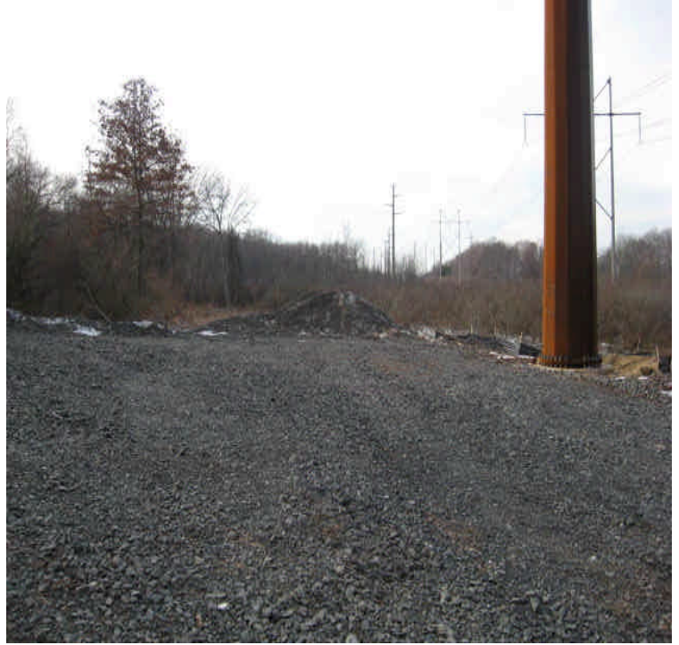
Tamarack Swamp Rd.: Snow and associated sediment had been plowed up to the boundary of the wetland. Snowmelt could result in the deposition of sediment.
