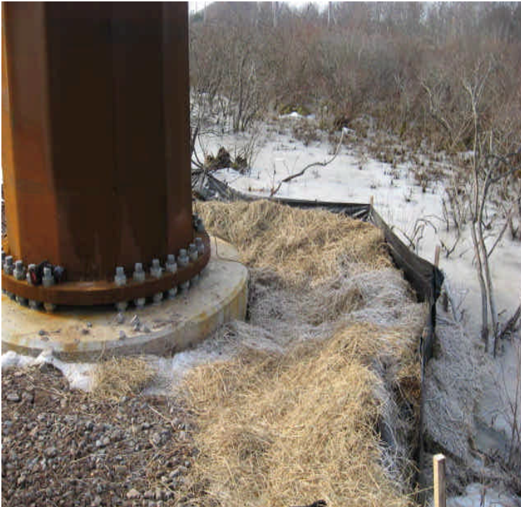
Tamarack Swamp Rd.: New controls were installed to encompass the soil after grounding crews had damaged the existing silt fence. Evaluate whether the activities here caused additional encroachment.
