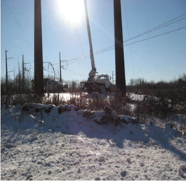
Carpenter Lane: Line work was underway from Beseck to Durham Rd.
