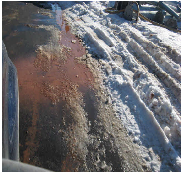
Old Farms Rd: Sediment tracking and turbid run-off noted from active areas.
