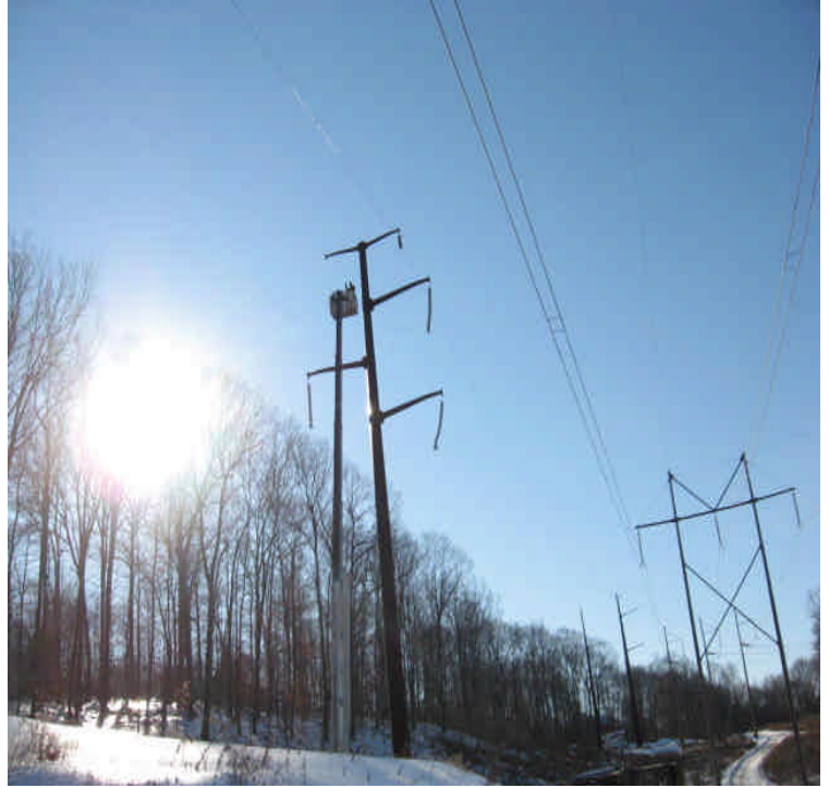
High Hill Rd: Line work underway.
