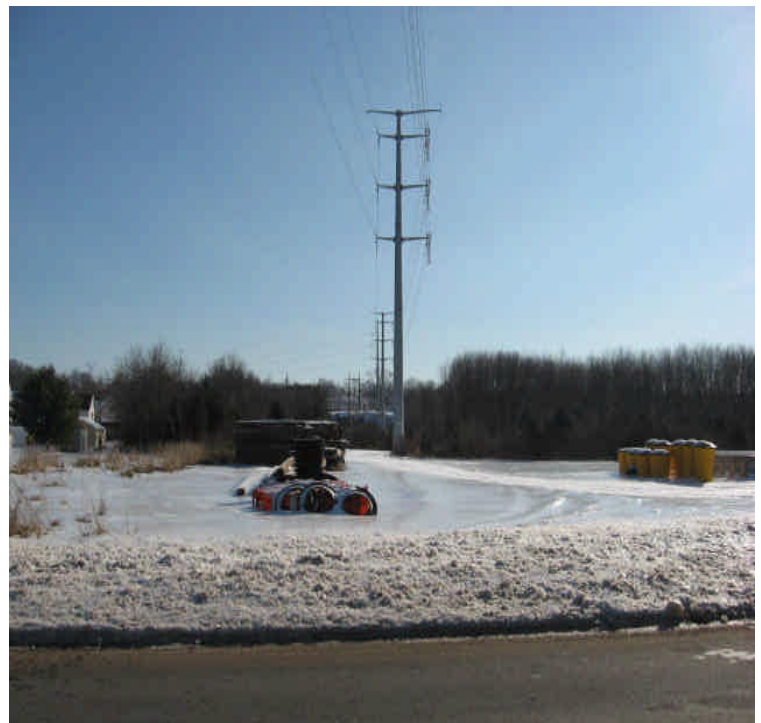
Pond Hill Rd: View of the previously disturbed area where the stockpile had been. Seed and mulch were applied prior to the snow cover.
