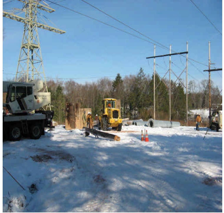
Old Farms Rd: Foundation and structure installation is underway.
