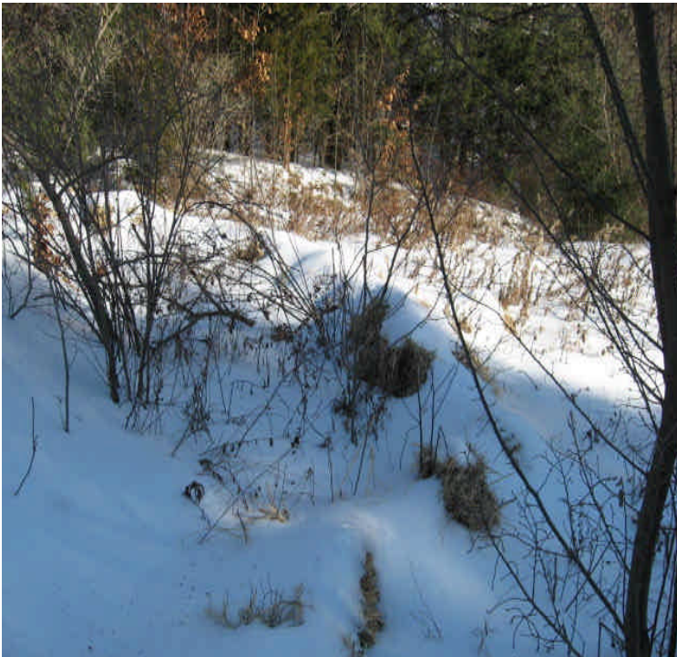
Old Farms Rd: Controls installed at the base of soil stockpiles prior to snow cover.
