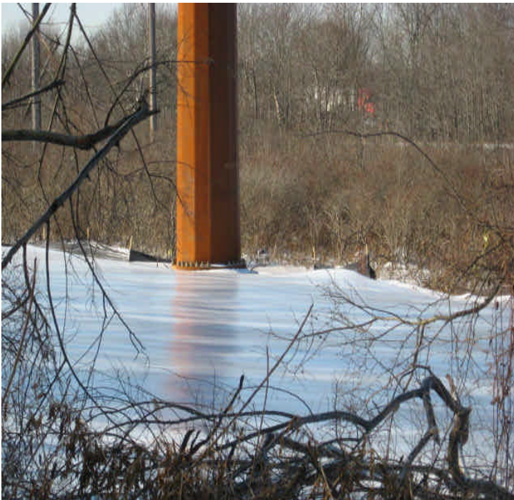
Tamarack Swamp Rd: Controls were degraded from grounding crew activities and are now under snow cover.
