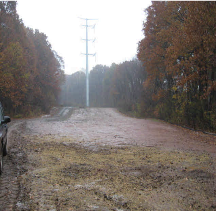
Docker Dr: View of the large disturbed area. Previously applied seed and mulch has washed away. Additional attention is needed here to stabilize the area for the winter months.
