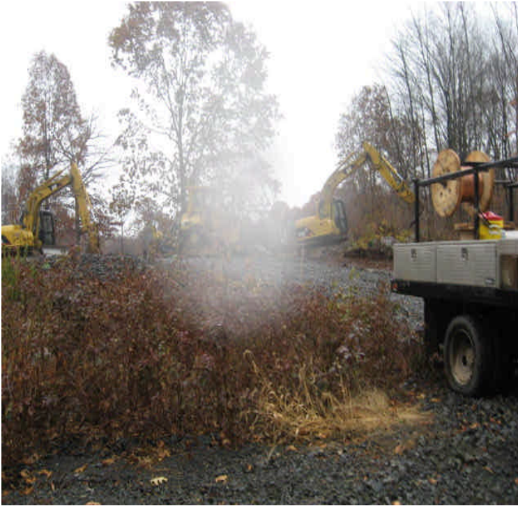
Durham Rd: Crews were installing grounding wires.
