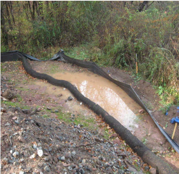
Docker Dr: Turbid run-off was pooling against controls. Previously applied mulch and seed has largely washed away in this area.
