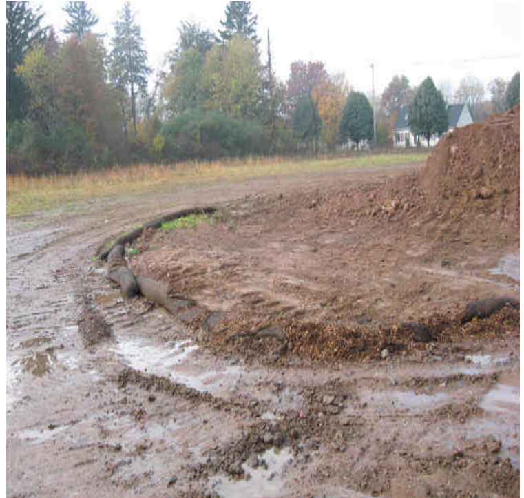
Pond Hill: Soil stockpiles from other sites are being stored here. Controls have been overwhelmed by sediment and vehicle traffic. Soil was being removed during the inspection.
