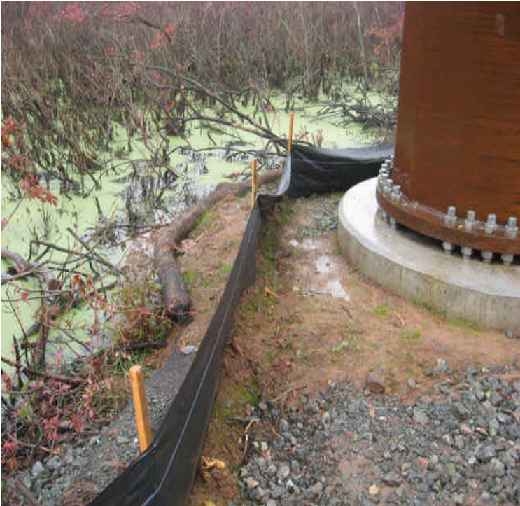
Tamarack Swamp Rd: The silt fence remains in place but the sediment that had been pushed beyond the original controls should be removed carefully.
