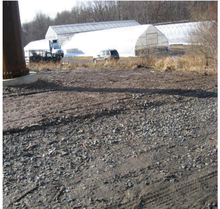
View of exposed pad area within the contractor yard. Begin stabilization within approved timelines.
