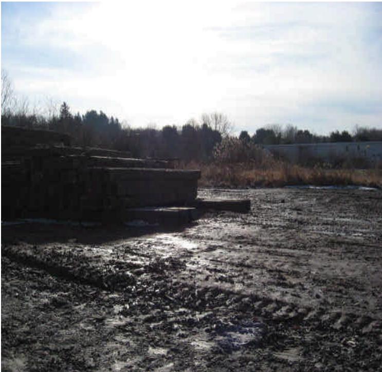
Timber mats stockpiled in an exposed area within the contractor yard. Begin stabilization within approved timelines.
