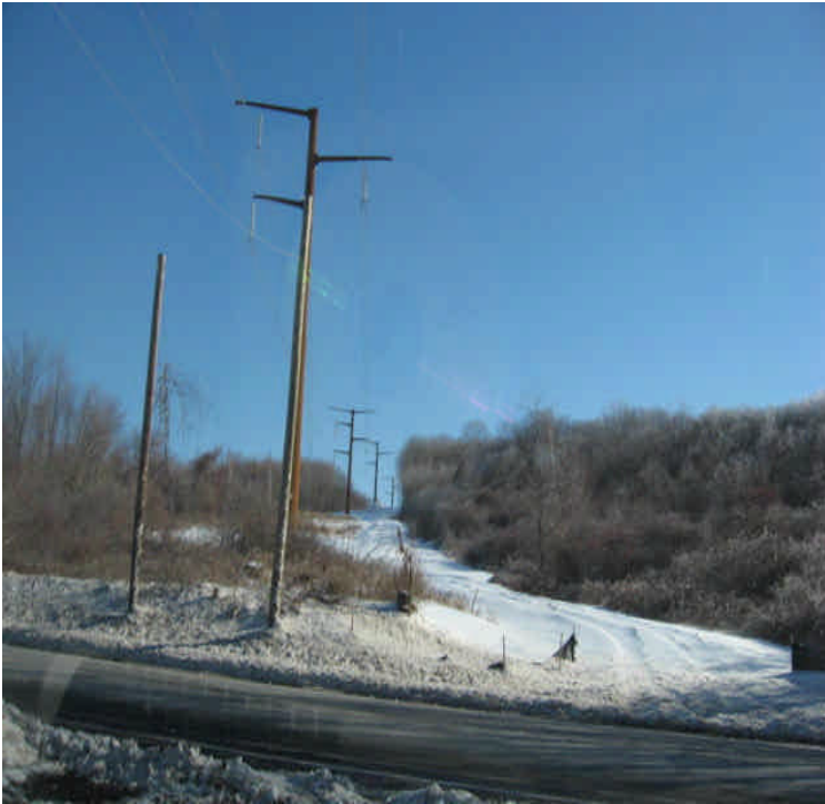
Entrance to the ROW off Rte. 17, looking to the east.
