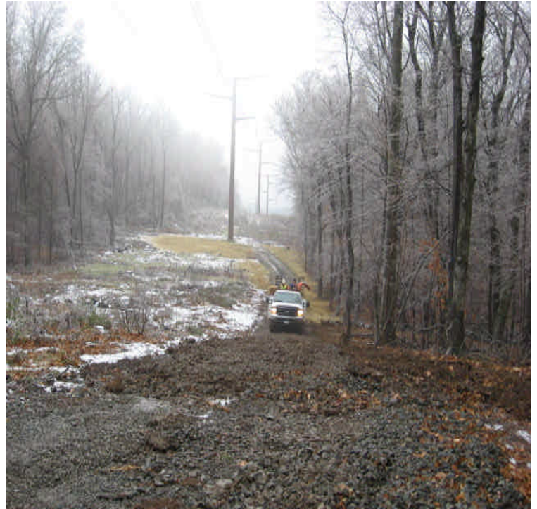
Reclaimed areas off Black Walnut Drive had been mulched and seeded.
