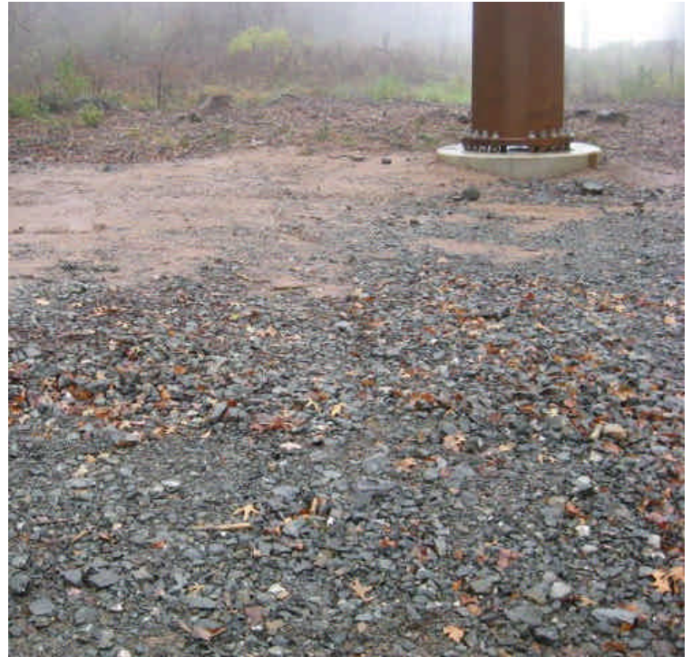
Stone from the pad is sinking into the soil and being covered over, adjacent to the no access area.
