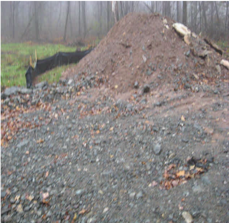
Soil stockpile off Black Walnut Drive with silt fence in place at it's base.
