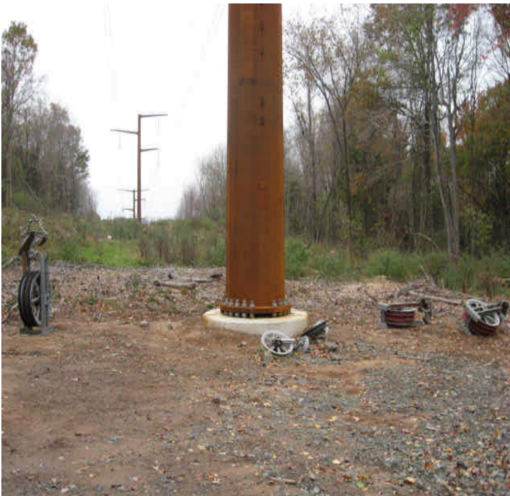
View of line pulling materials.
