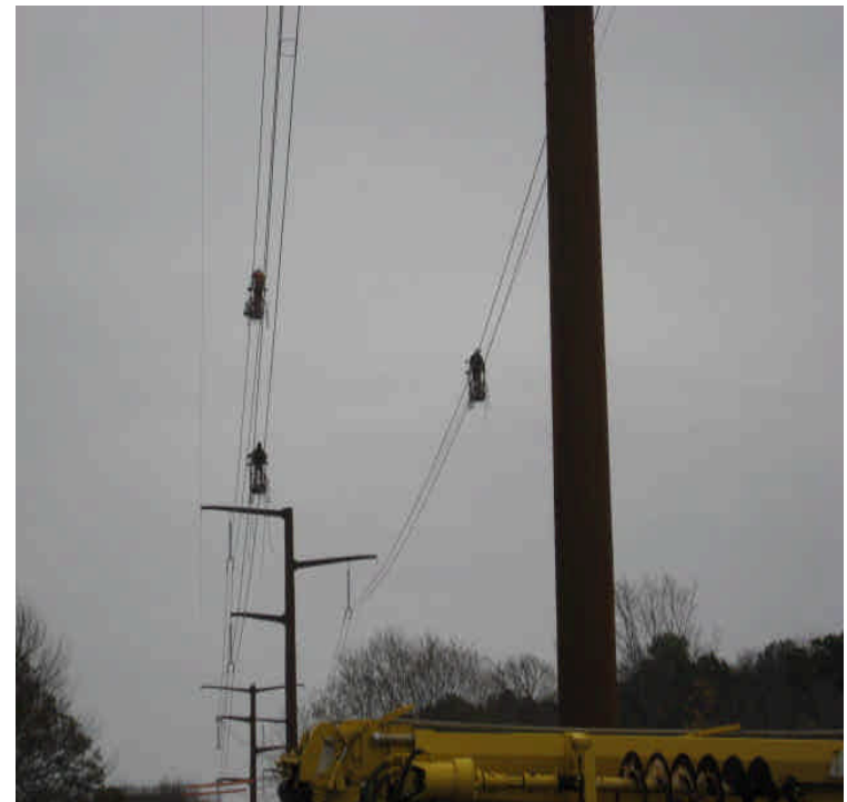
Line work underway near the contractor receiving yard.
