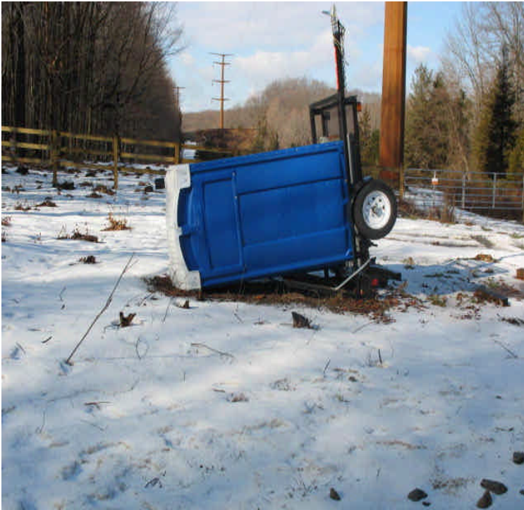
Arbutus St: Sanitary facility remains tipped over but crews are on break.
