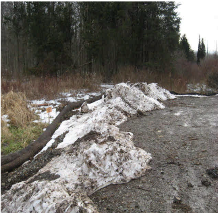
Carpenter Ln: Snow stockpile located at controls adjacent to the wetland. Use caution and observe wetland boundaries when plowing snow in order to keep snow and sediment contained.
