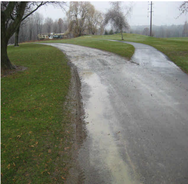
Durham Rd Golf Course: Turbid run-off noted coming from work and running along pave paths within the golf course. Attempt to control turbidity at the source.
