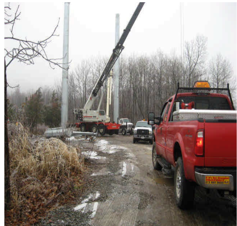
South of East Main St.: Pole installation was underway.
