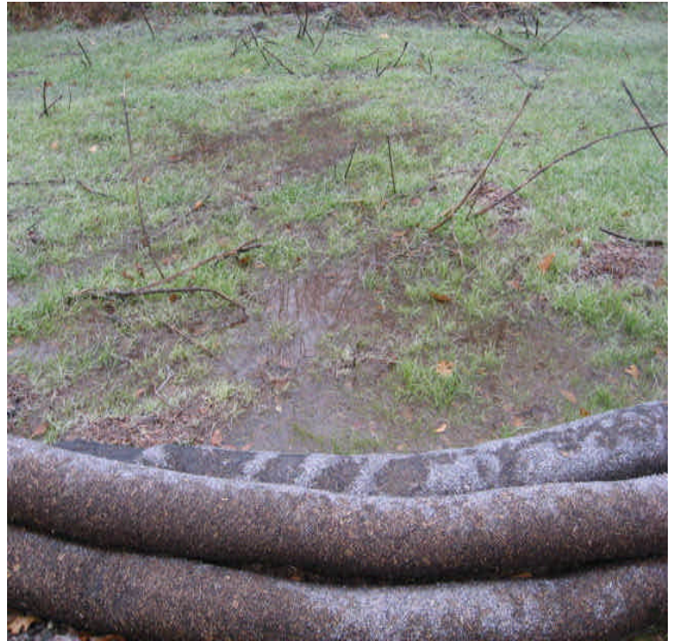
N. of Beseck SS: Water bars have been installed along access roads to divert stormwater to stable areas. Turbid water was not noted within the wetlands since installation.
