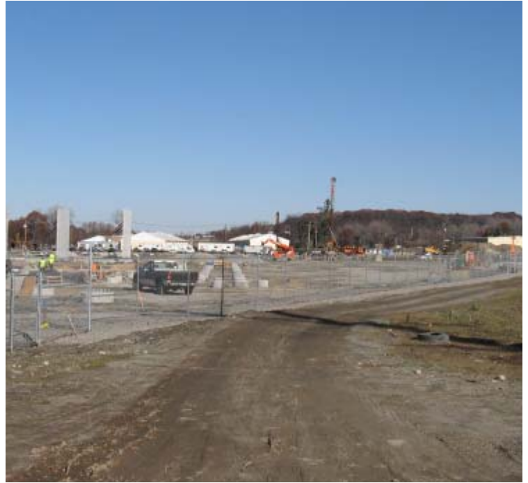
East Devon Substation: An additional view of the construction at the substation.
