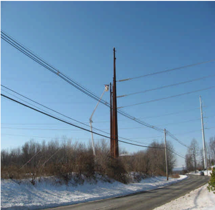
Line work from Segment 2A into the switching station.
