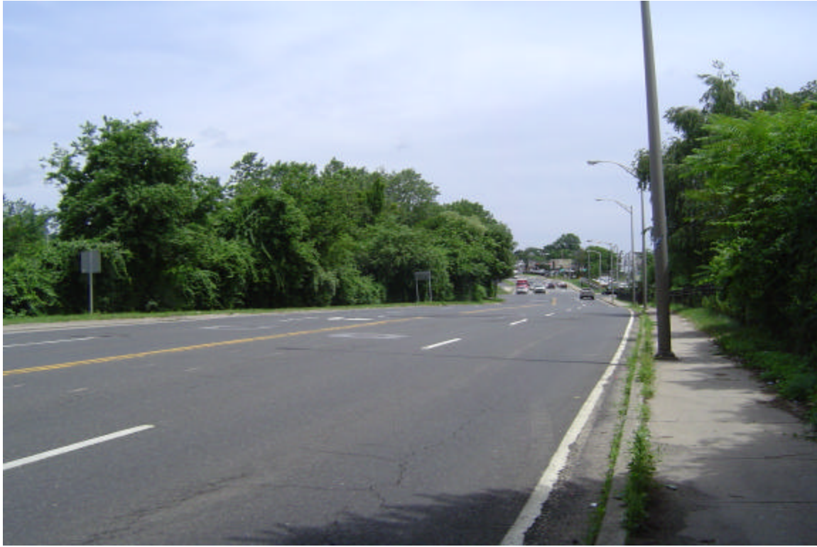
Photo 3: Route 123 (New Canaan Avenue) at the Route 7 overpass looking eastbound.
