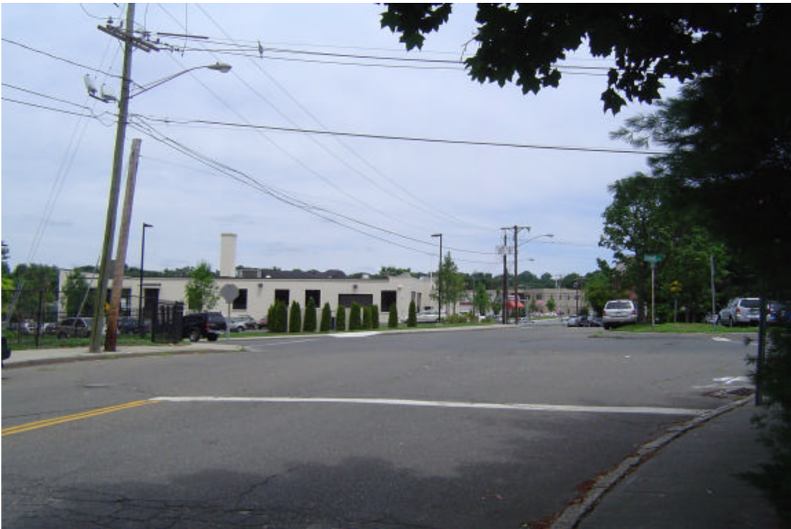
Photo 6: Tindall Avenue, looking eastbound at intersection with Grand Street and proposed transmission line route from Grand Street to Private and CL&P property.
