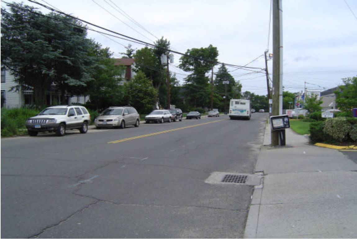
Photo 9: Route 123 (Main Street) between Catherine Street and Holmes Street, looking southbound.
