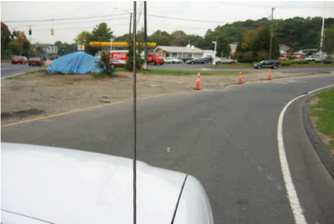
Photo on the shows the Rt 107/7 intersection. Some areas have been seeded/mulched but final restoration is still required. Sedimentation to the roadway is noted. 10/04/06
