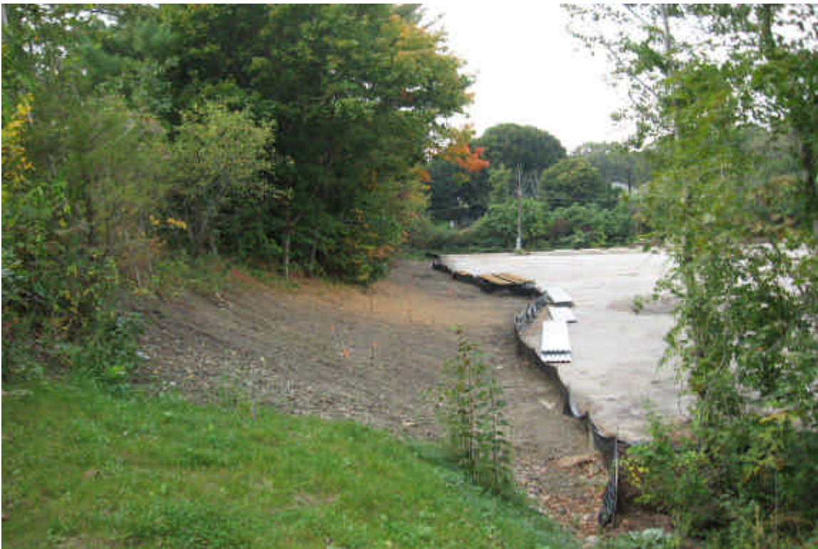
Photo shows a view of the silt fence installed at the Gilbert & Bennett lot. Seed and mulch are still needed here along the slope. 10/04/06
