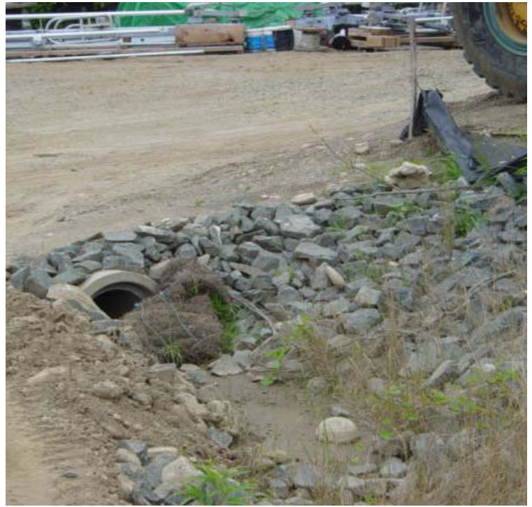
Norwalk Junction: Photo on the left shows the ongoing work on foundations and structures at the station yard. Photo on the right shows sediment accumulation remaining in the swales on site. This should be removed and the haybales need to be replaced. 7/26/06
