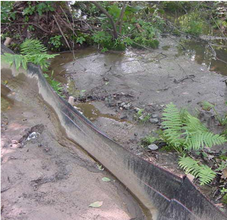
Archers Lane: Photo on the left shows the area along the silt fence at the 1 st wetland crossing where accumulated sediment remains in the wetland. Contractors are being scheduled to remove this but more final stabilization measures will be needed. Photo on the right shows an overview of the work and structures in the station yard. 7/26/06.
