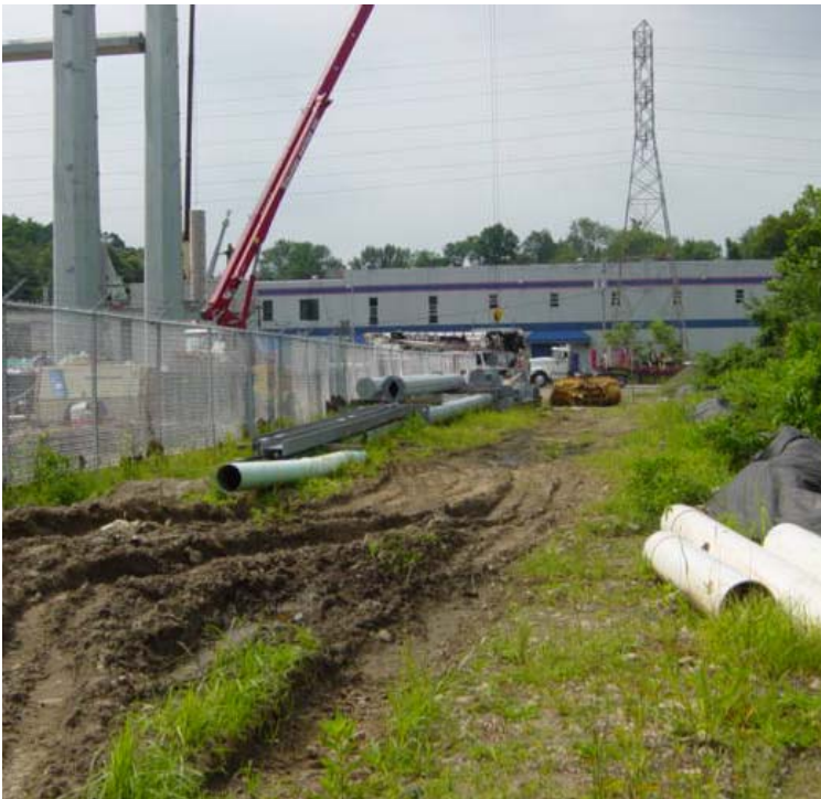
Norwalk Junction: Photo on the left shows where some vehicle traffic caused significant ruts in the soil. This area needs to be smoothed out/restored and mats or plates should be used here to reduce disturbance. Photo on the right shows the plate in place across the swale for vehicle access. 7/26/06.
