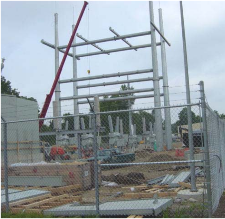
Norwalk Junction: Photo on the left shows the ongoing work on foundations and structures at the station yard. Photo on the right shows sediment accumulation remaining in the swales on site. This should be removed and the haybales need to be replaced. 7/26/06
