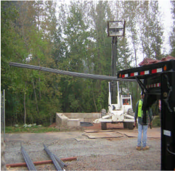
Additional photographs of the work associated with the 345 kV Turning Structure: Photo on the left shows rebar being transported to work area. Photo on the right shows approximate location of caisson drilling. 10/5/05
