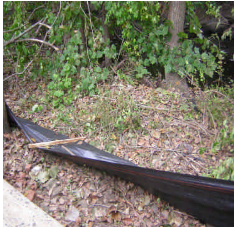
The silt fence behind the jersey barriers and adjacent to the river was in need of repair. Contractors were aware of the damage and were preparing for repairs. 10/5/05
