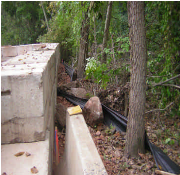
The silt fence behind the jersey barriers and adjacent to the river was in need of repair. Contractors were aware of the damage and were preparing for repairs. 10/5/05
