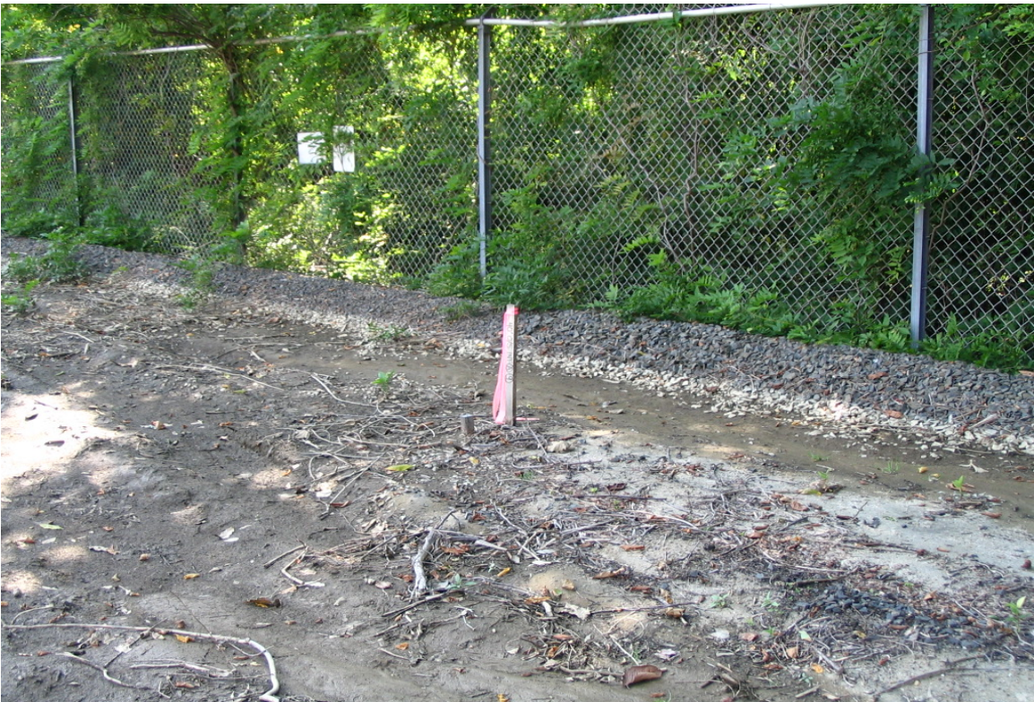
View of the line (lighter color) along the perimeter stone berm where the rain water had reached. The site was muddy but there were no discharges to the adjacent wetlands. 9/23/04
