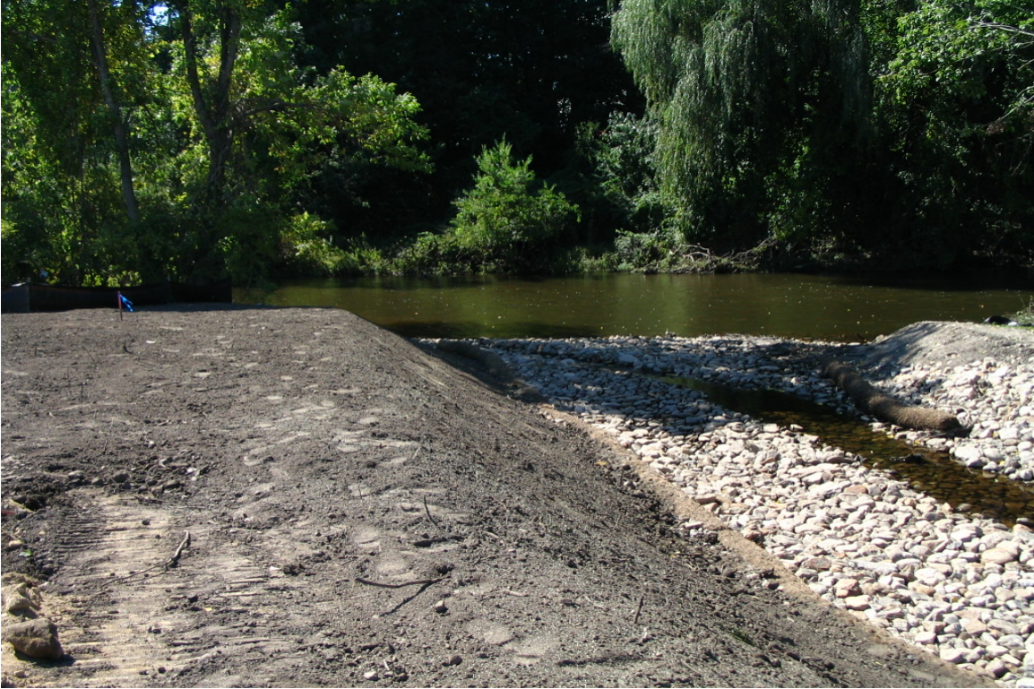
Portions of the soil placed on the overflow channel had been washed away during the high flows caused by Hurricane Ivan before vegetation could establish. The remaining soil was raked into place and reseeded 9/23/04
