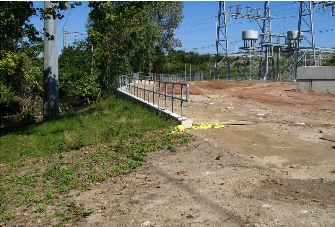
View of the area scoured in the spring which did not erode despite the floodwaters that came over the area. The vegetation was established enough to hold the soil. 9/23/04
