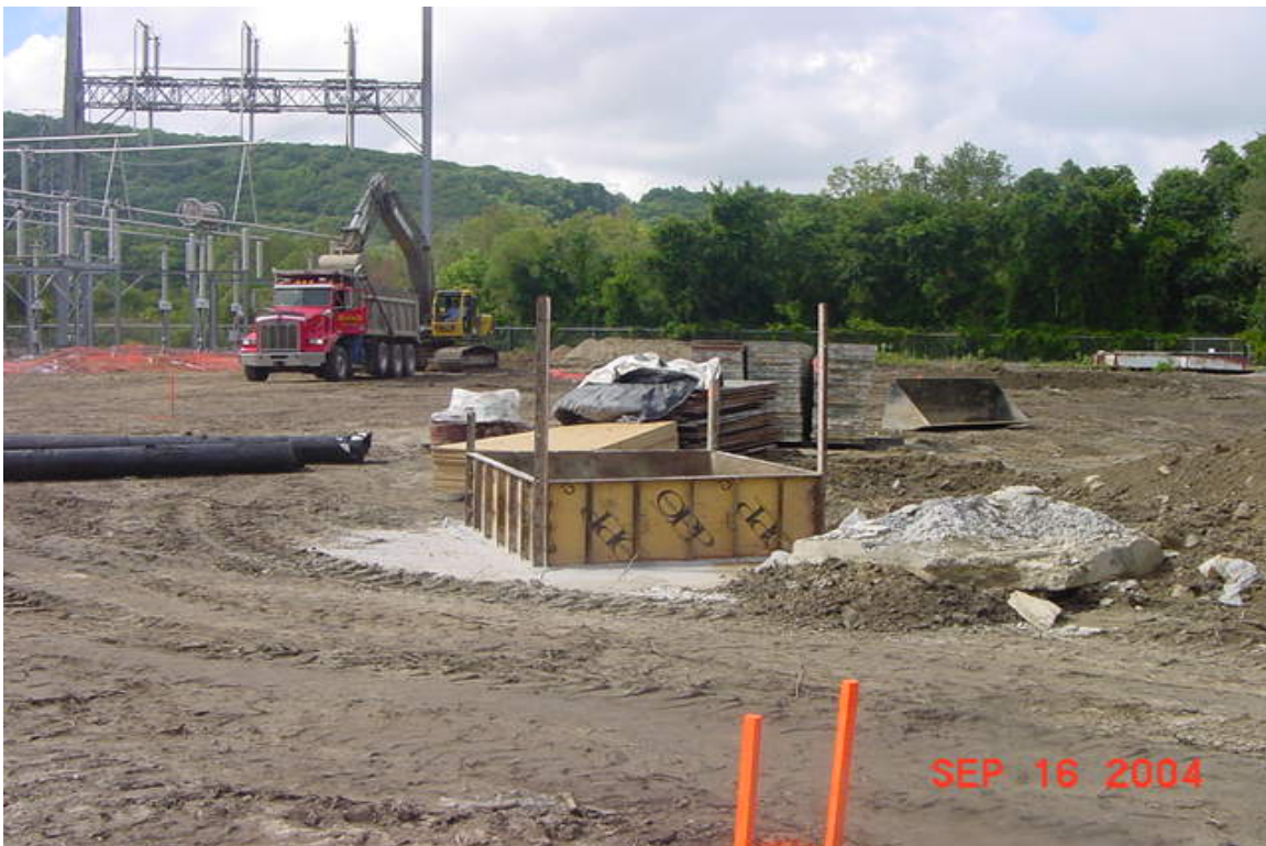
Overall view of the yard including the concrete washout station and soil being loaded into a truck to be hauled off site. 9/16/04
