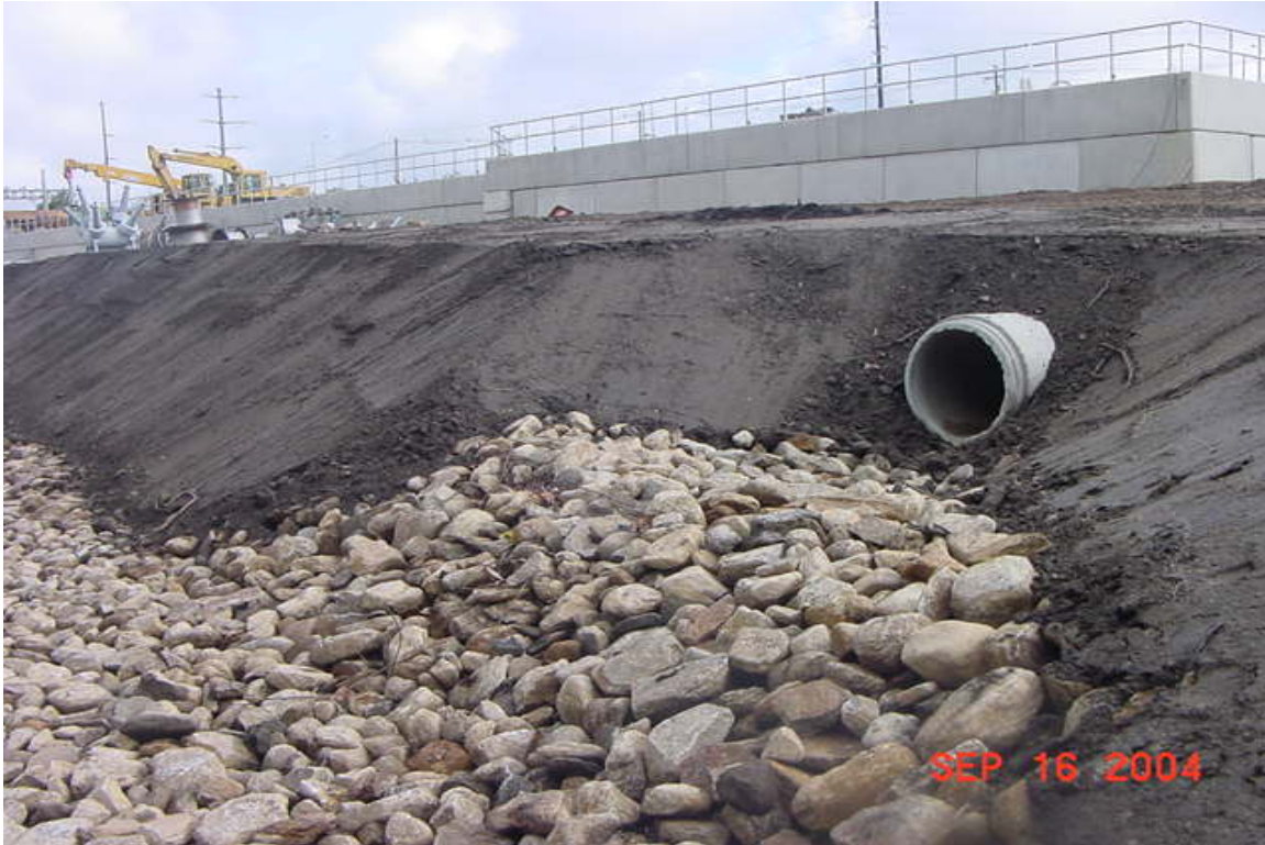
View of the outlet at the overflow channel following placement of topsoil. The catch basin inlet to this pipe is not yet at grade or active. 9/16/04
