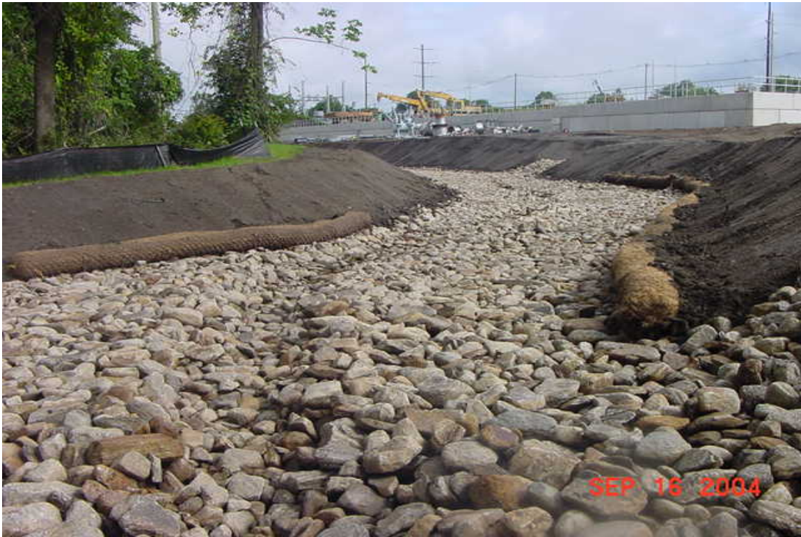
View of the overflow channel following placement of topsoil and seed on the sides and banks of the channel. The biologs remain in place here. 9/16/04
