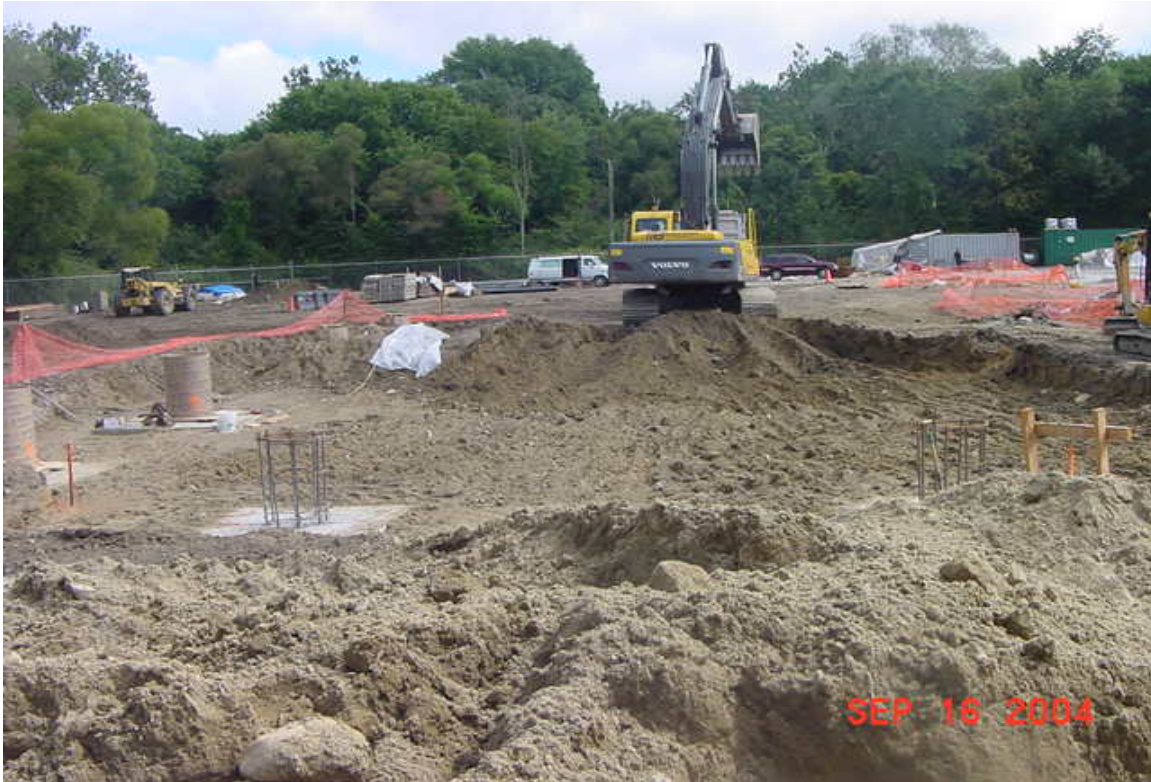
Plumtree Substation: View of the excavation for the GIS concrete pad. Soil is being hauled off site and the remainder is being stockpiled. 9/16/04
