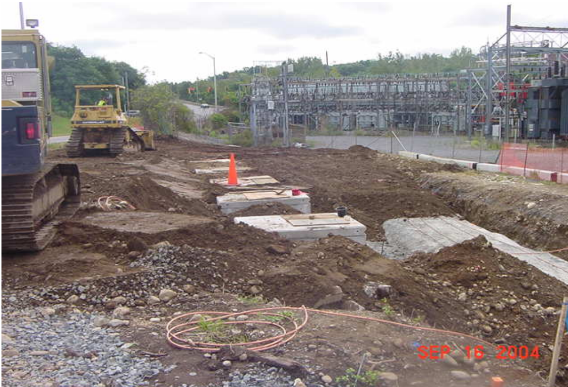
View of form footings near the control building. The conduit bank has also been covered in concrete and are being backfilled. 9/16/04
