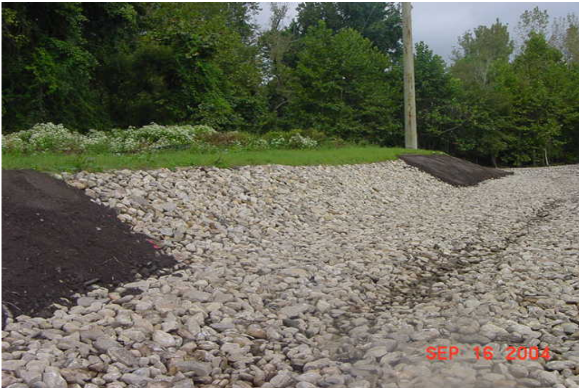
Portions of the channel will remain with bare stone as according to the approved plans. 9/16/04
