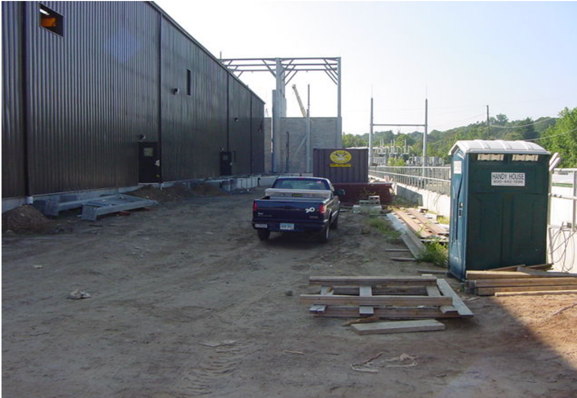
Work on the concrete cable boxes/trays continues around the GIS building while cable is being pulled within the yard. (9/1/05)
