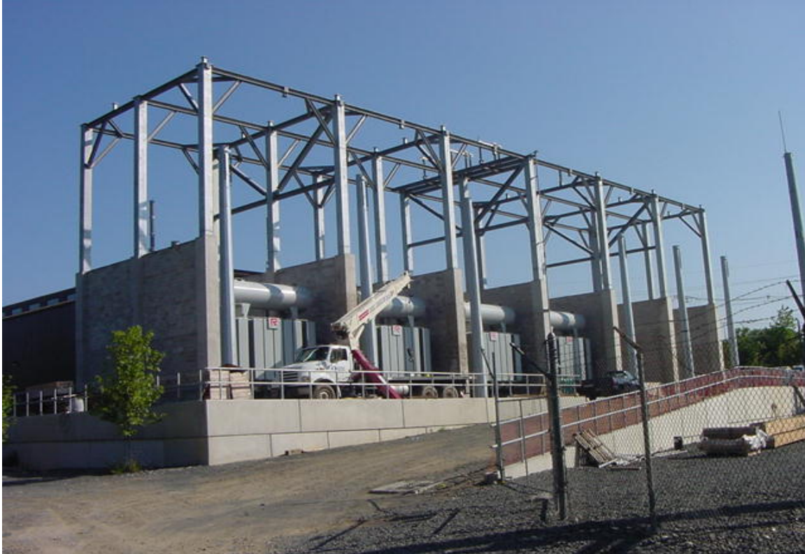
Norwalk Substation: Work continues on the transformers and equipment adjacent to the GIS building. (9/1/05)
