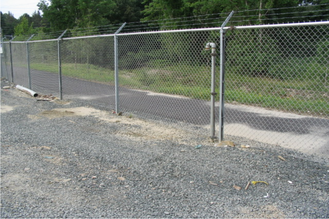
The yard has some slight sedimentation on to the bike path from the access road. The stone berm should be continued to help keep sediment on site. (8/19/05)
