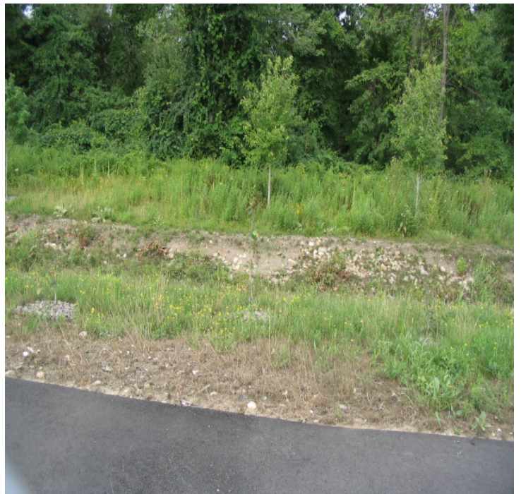
View of several areas along the overflow channel where vegetation has not returned sufficiently. The slopes will be reseeded following the dry period of the summer to ensure better results. (8/19/05)
