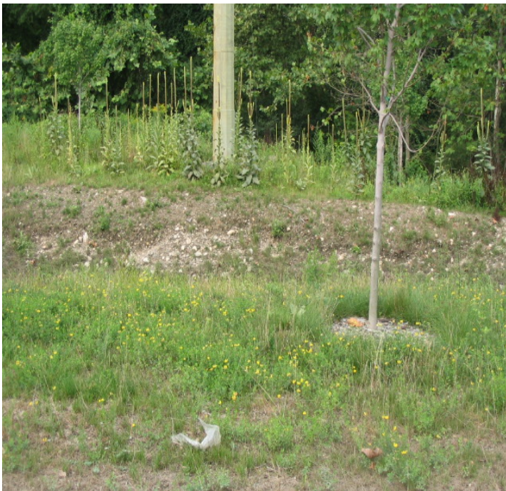
View of several areas along the overflow channel where vegetation has not returned sufficiently. The slopes will be reseeded following the dry period of the summer to ensure better results. (8/19/05)
