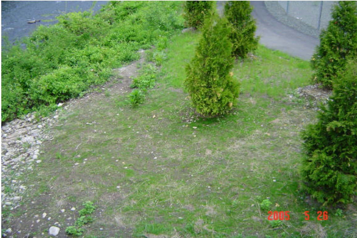
Norwalk Substation-Vegetation is increasing at the bank of the river where DOT had recently performed their work. (5/26/05)
