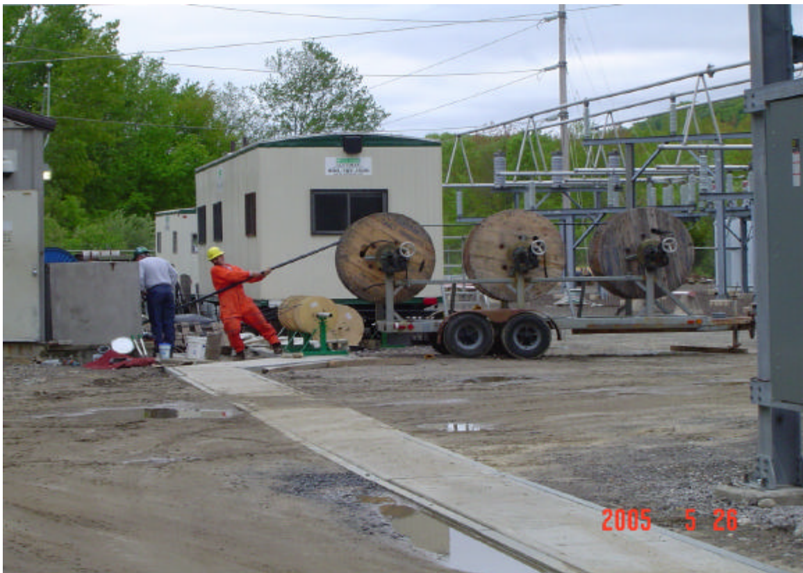
Active cable pulling is occurring in several locations throughout the site. (5/26/05)
