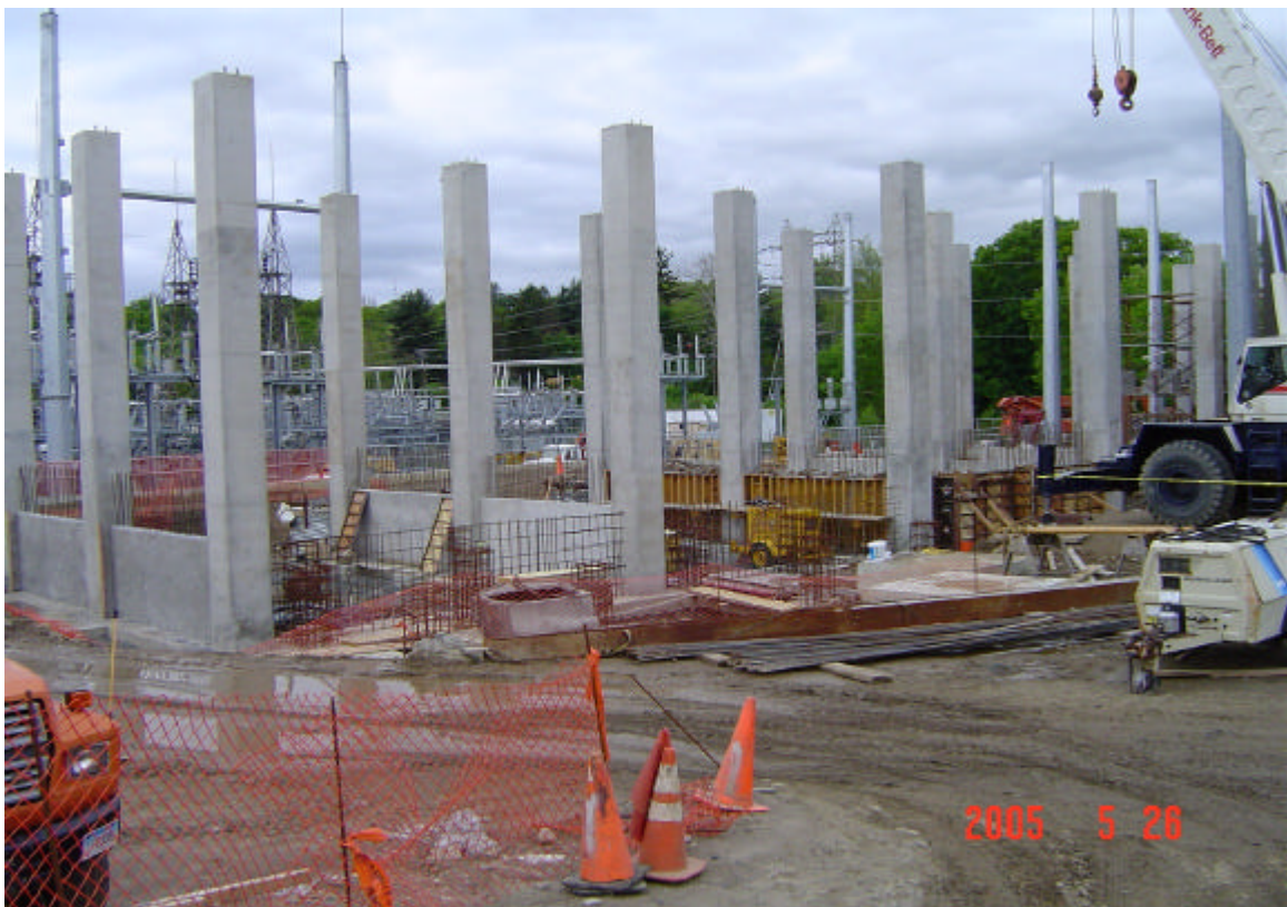
View of the foundation and structure work near the GIS building and retaining wall #3. (5/26/05)
