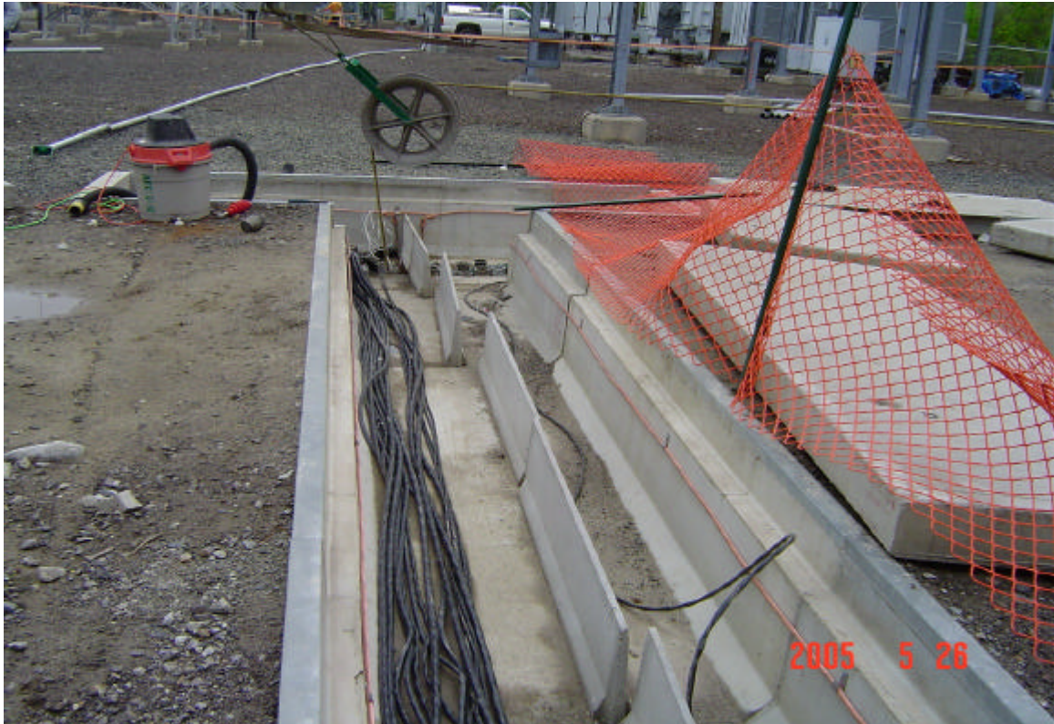
Plumtree Substation- Cable is being pulled in the trenches surrounding the slab. (5/26/05)
