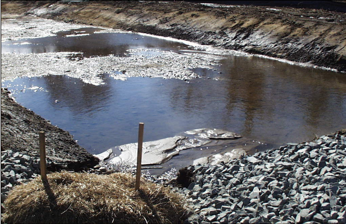
A VIEW OF THE SEDIMENT BASIN. THE DEWATERING DISCHARGE REMAINS CLEAR AND IS DIRECTED TO THE BASIN. A SMALL AMOUNT OF EROSION OCCURRED ALONG THE SWALE AND INTO THE BASIN. 2/27/04
