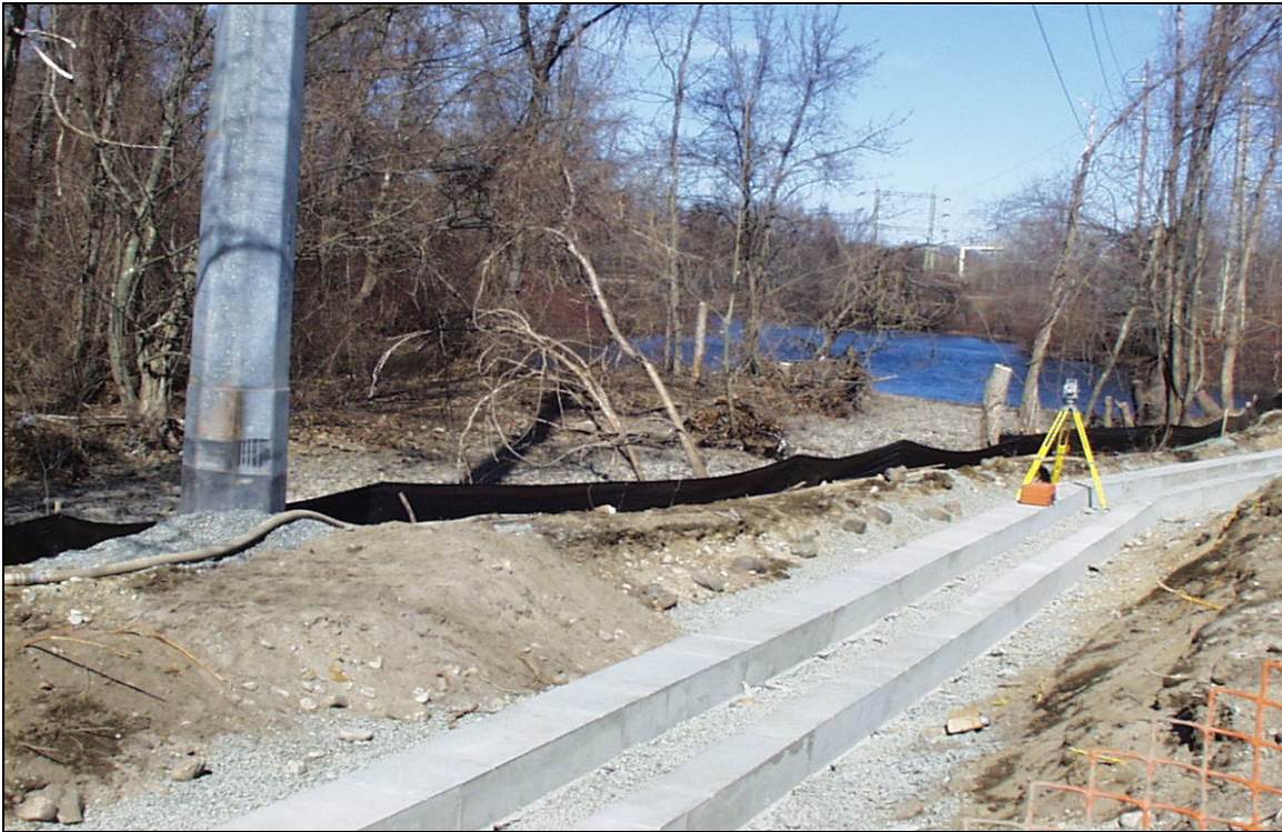
VIEW OF THE NEW RETAINING WALL FOUNDATION. THIS AREA IS WHERE DISCUSSIONS ARE ONGOING, REGARDING ADDITIONAL FUTURE BANK STABILIZATION ALTERNATIVES 2/27/04
