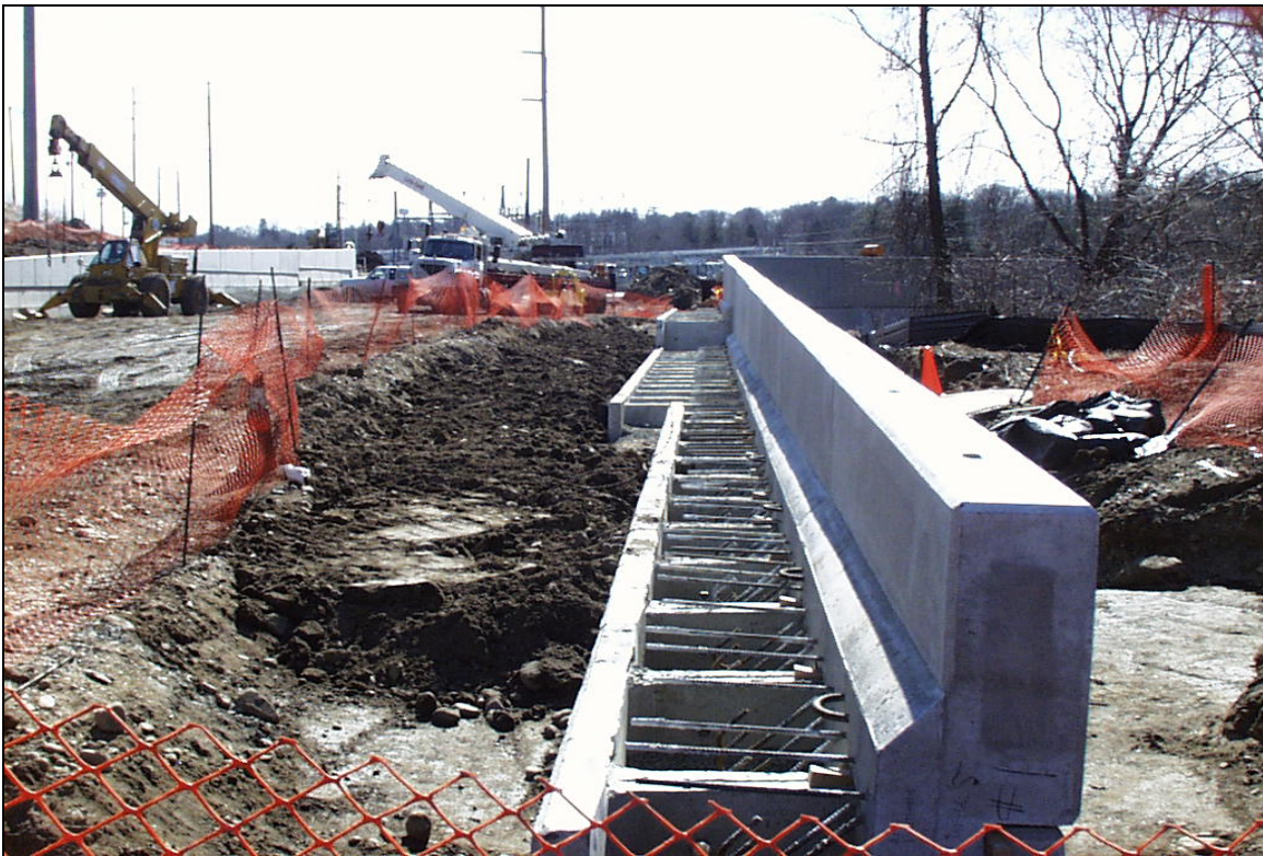
VIEW OF THE NEW RETAINING WALL FOUNDATION. THIS AREA IS WHERE DISCUSSIONS ARE ONGOING, REGARDING ADDITIONAL FUTURE BANK STABILIZATION ALTERNATIVES 2/27/04
