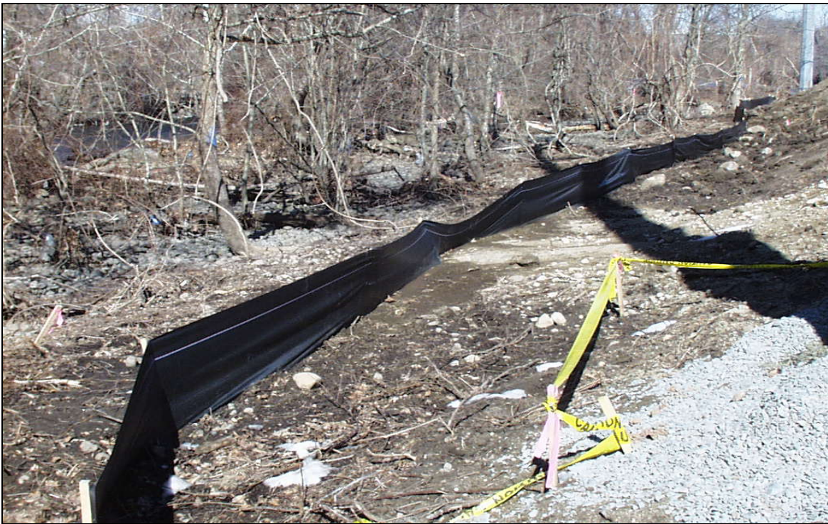
THE SNOW COVER IS GONE FOR THE MOST PART AND RAINS COULD BRING STRESS TO THE SILT FENCE. A SECOND BARRIER SHOULD BE INSTALLED AT THE BASE OF THE STOCKPILE 2/27/04
