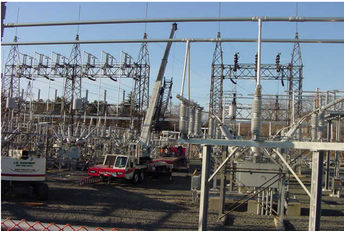
Norwalk Substation: Structures were being removed from the electrified yard. 1/26/06.
